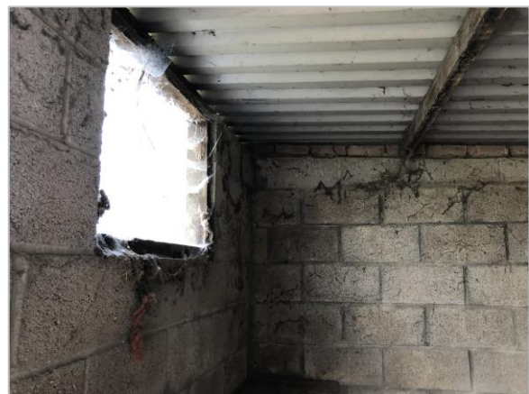
Photo 6 Internals of southern part of building
