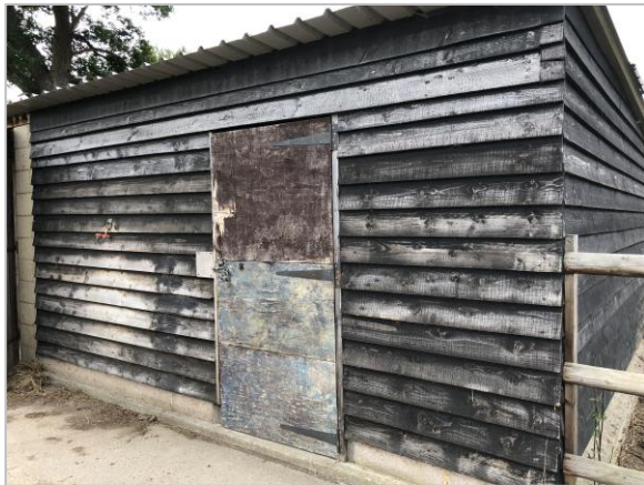
Photo 9 Cladding to northern part of building
