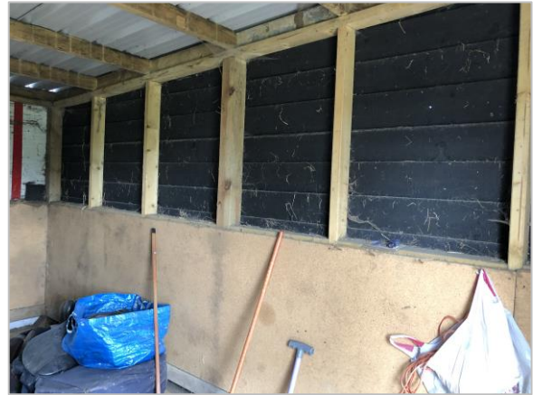
Photo 8 Internals of northern part of building
