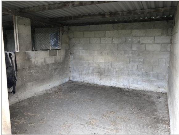
Photo 7 Internals of southern part of building
