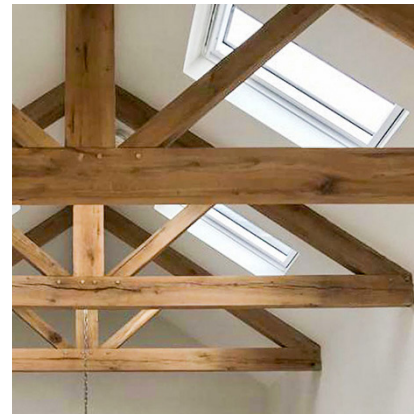
Exposed timber trusses
