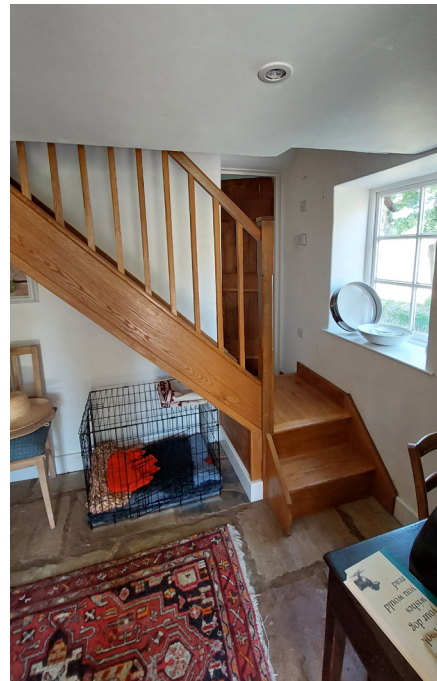
Figure 9 - Window to be adapted to form a new opening to the proposed extension, staircase to be adapted to create a more generous landing and bathroom door to be blocked and relocated
