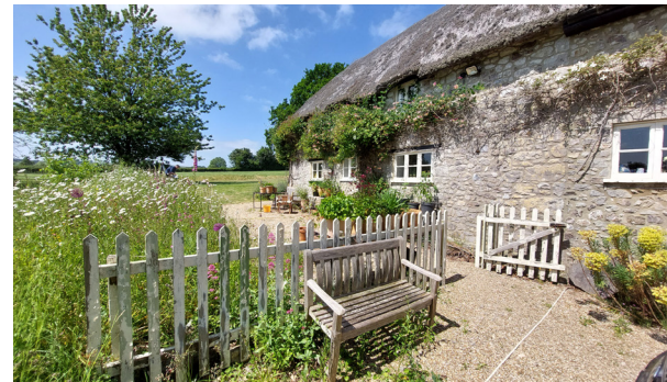
Figure 5 - South East Elevation
