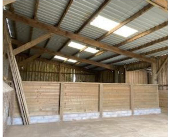
Photo 4: Internal view of the barn showing light from roof.
