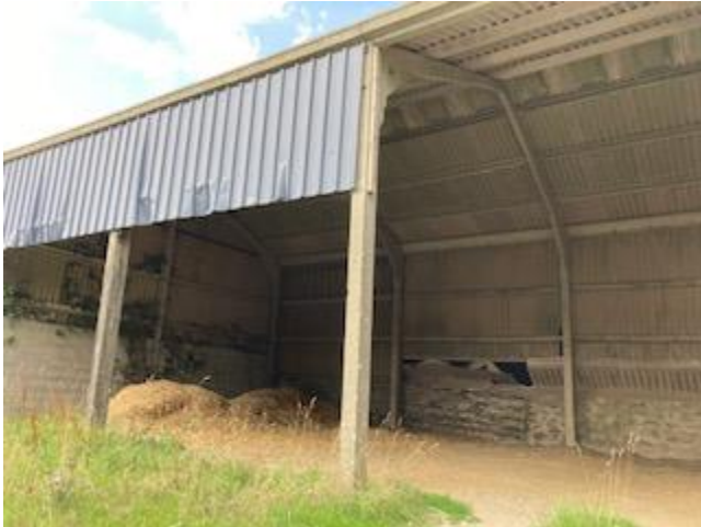
Photo 3: Open southern elevation of the barn.
