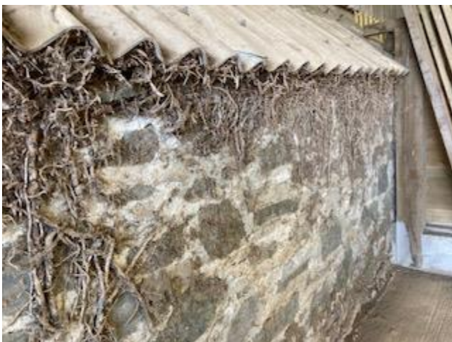
Photo 5: Sealed internal wall.
