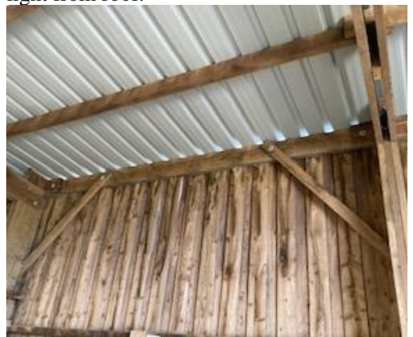
Photo 6: Internal timber cladded wall and new corrugated roof.
