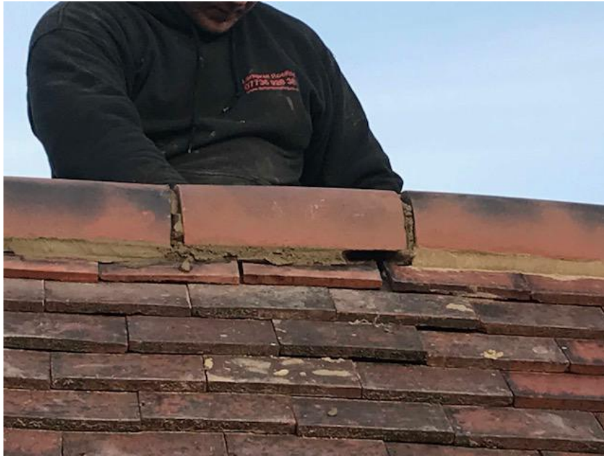
Photo 1: Example of ridge feature for pipistrelle
