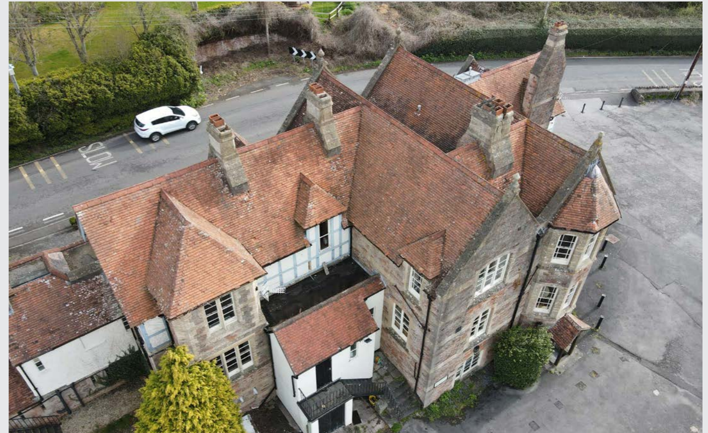
Drone photographs from the south elevation of the existing building
