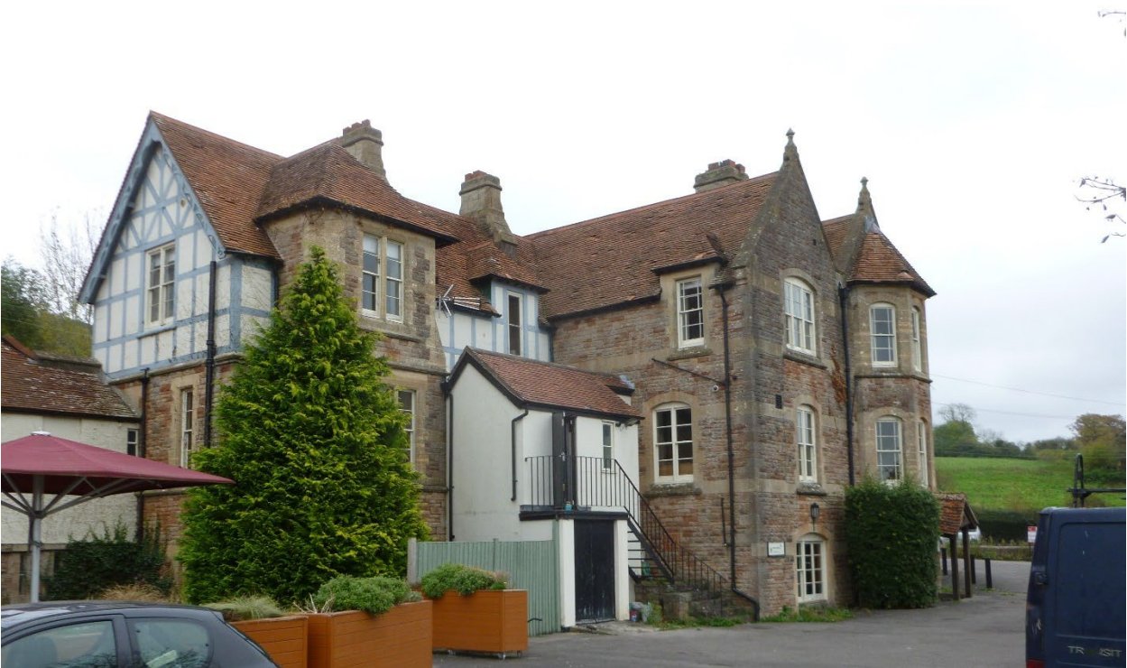
Plate 4: The public house element over three storeys, from the west
