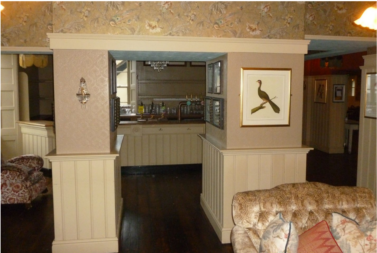
Plate 5: Former hearth opened out in PH upper ground floor
