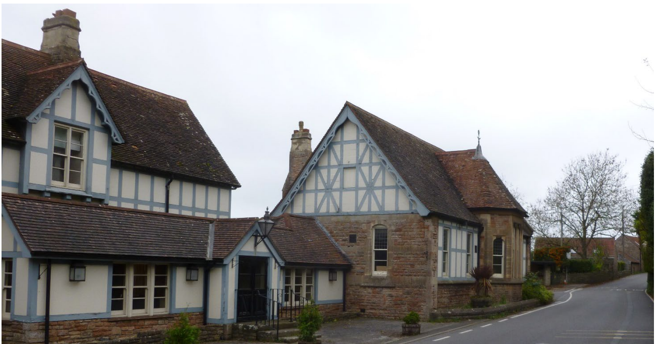
Plate 6: West end of the PH and connecting frontage element with the hall to the west
