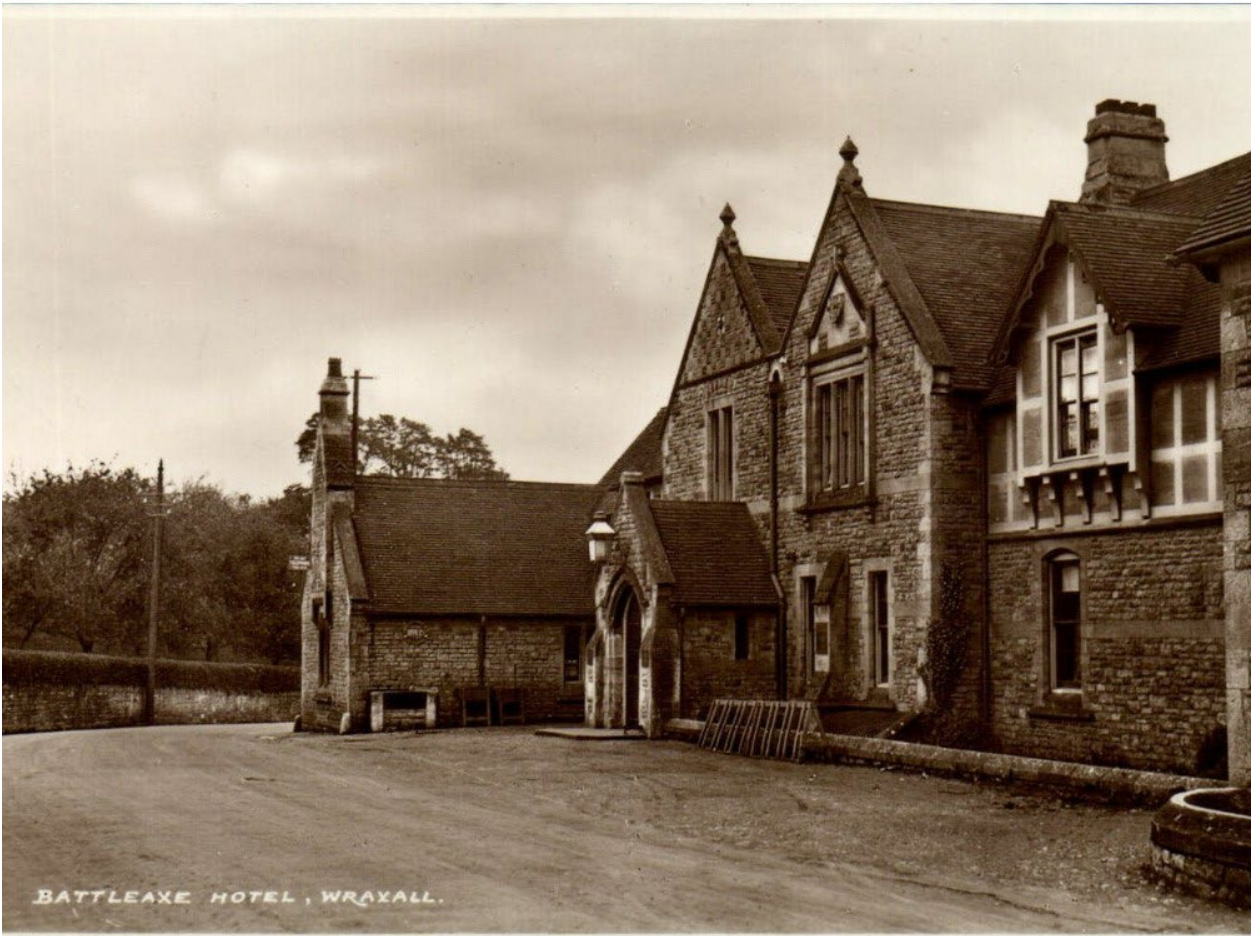
Figure 12: North elevation of the PH showing the extended early C20th eastern wing
