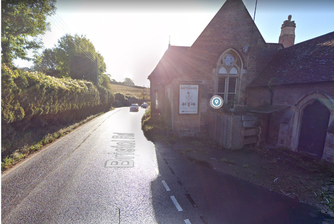
Plate A – Bristol Road Looking South
