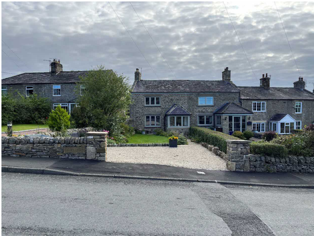
View of new access and parking area viewed from opposite footpath
