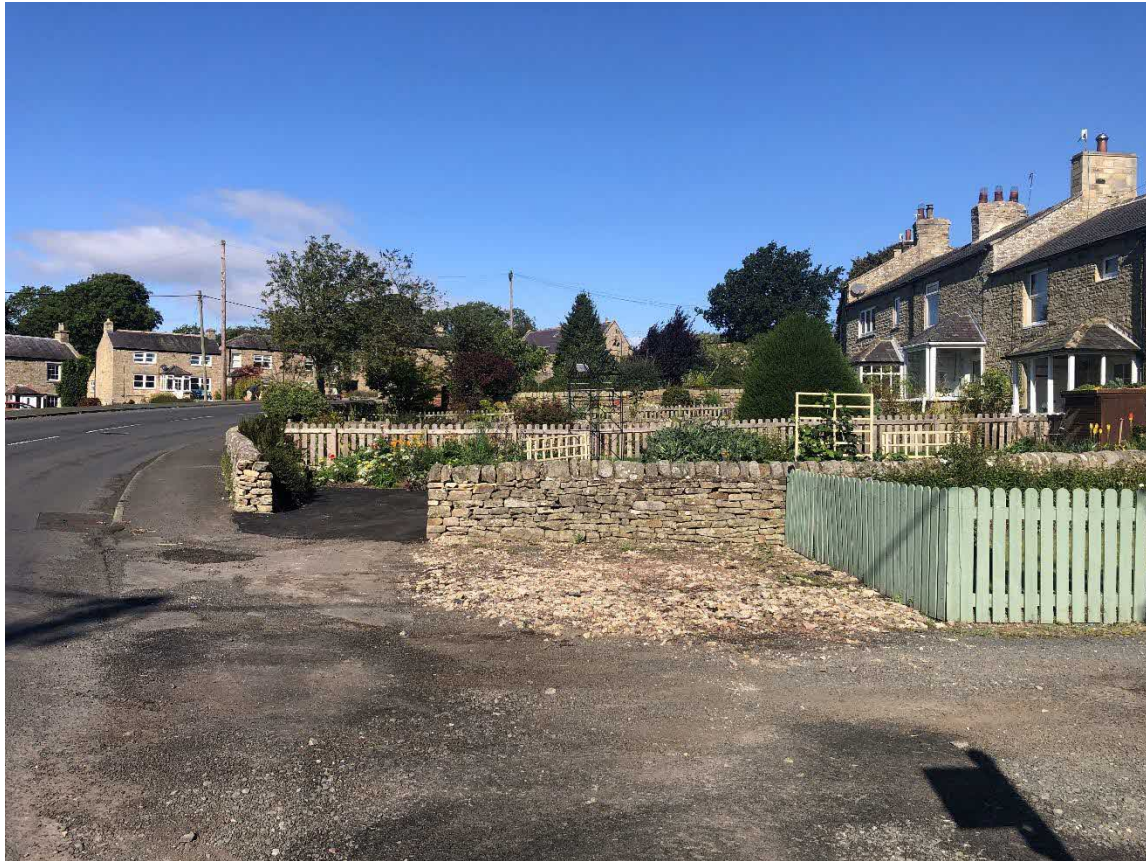
2no. domestic properties access on inner curve of main highway at southern end of terrace
