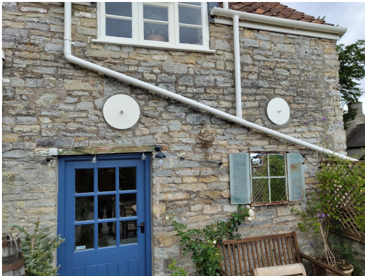
Photo showing North Wall of the Annex.
