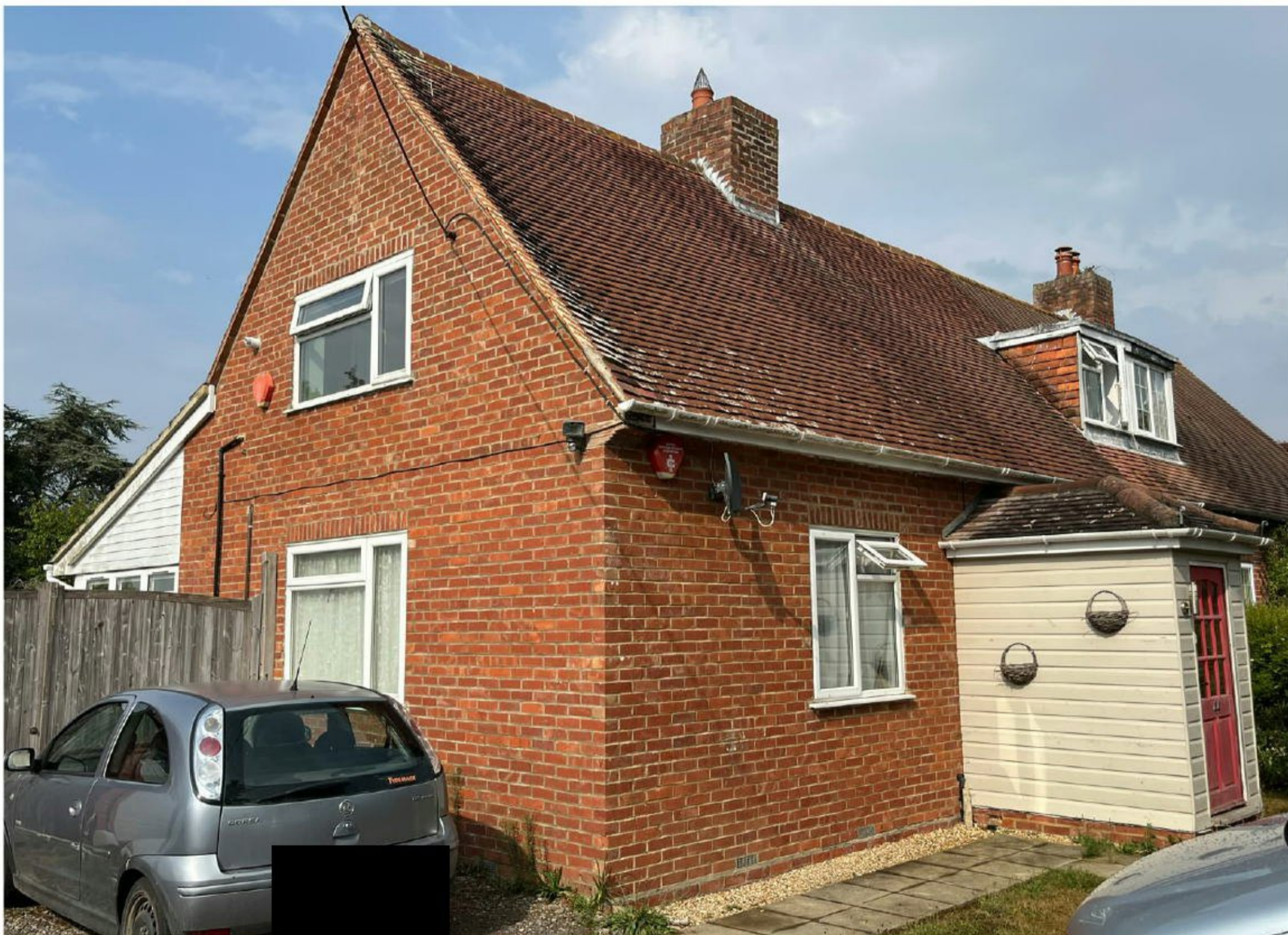
Gable to No 44
