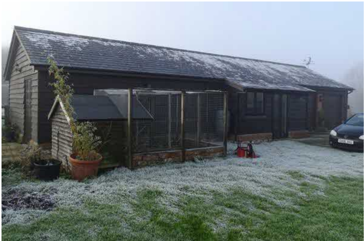
Image 13 – Building two – North/East facing elevation of the building
