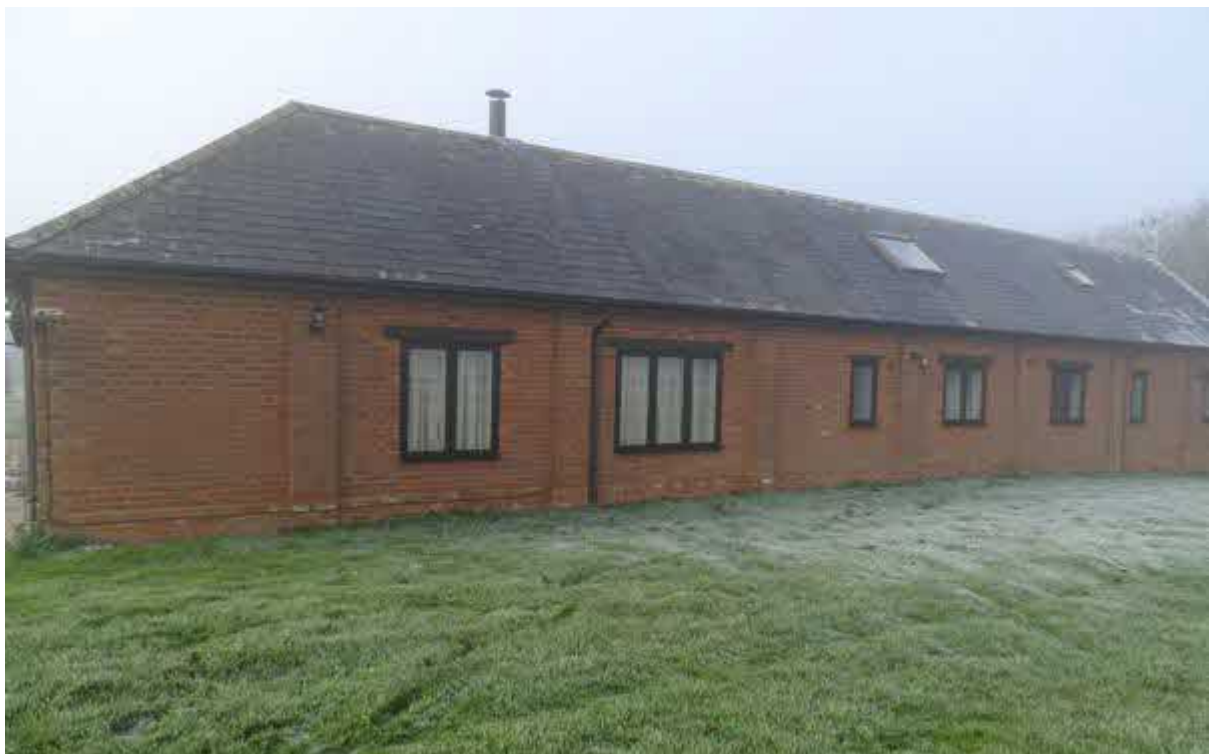
Image 8 – Building one – North/East facing elevation of the building
