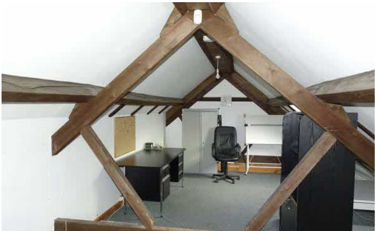
Image 12 – Building one – Internal view from within the building below the roof areas which offer a covered vaulted ceiling
