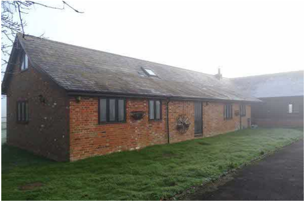
Image 7 – Building one – South/West facing elevation of the building
