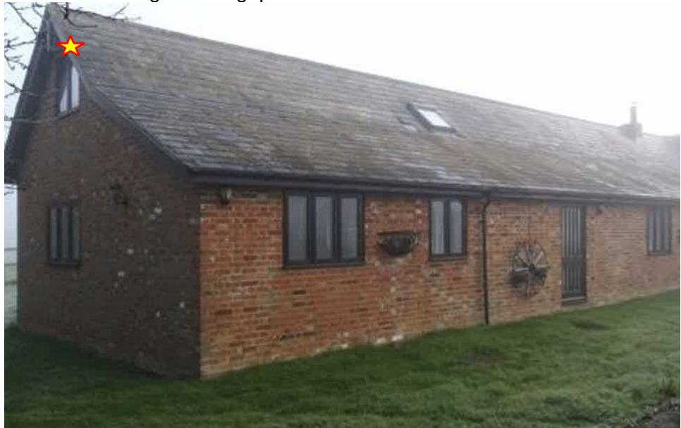
Roost 2 – Emerged from gap between the brickworks and soffit
