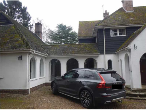
5. Central part of north elevation showing link
