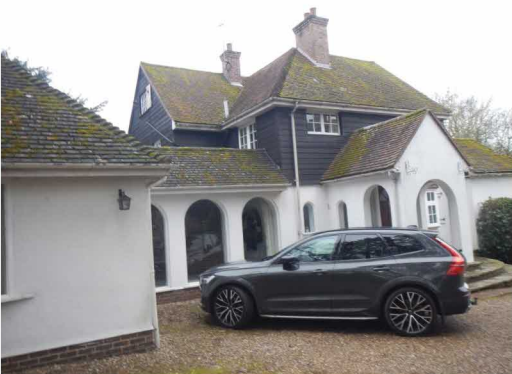
7. North elevation showing existing porch, two storey
