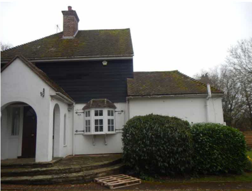
4. West end of North elevation
