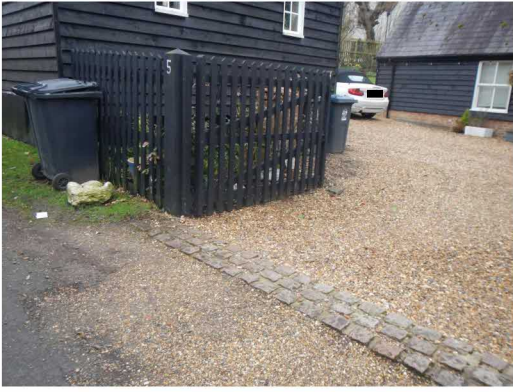
29. Existing gate to the vehicular access of 5 Fleece
