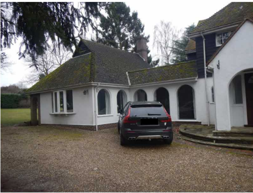
6. East end of North elevation
