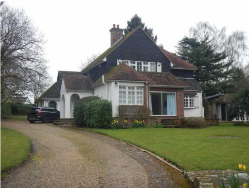
10. West elevation from site access
