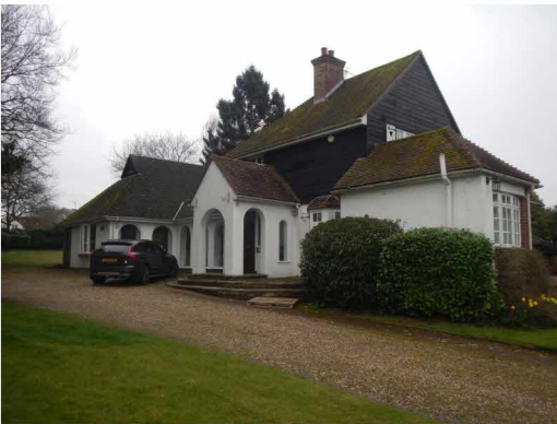
3. North elevation from within the site
