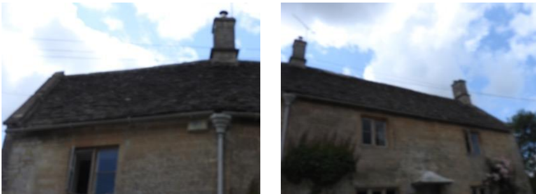
Figs. 7 & 8 Ridges and roof tiles to the front
