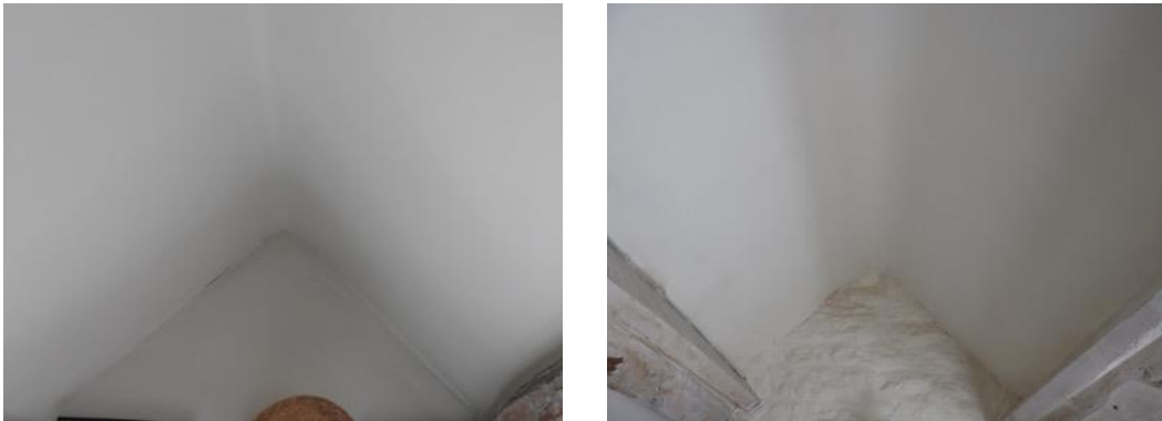
Fig. 19 Vaulted roof voids
