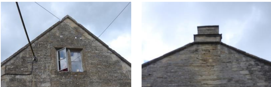
Figs. 15 & 16 Sealed Gable ends
