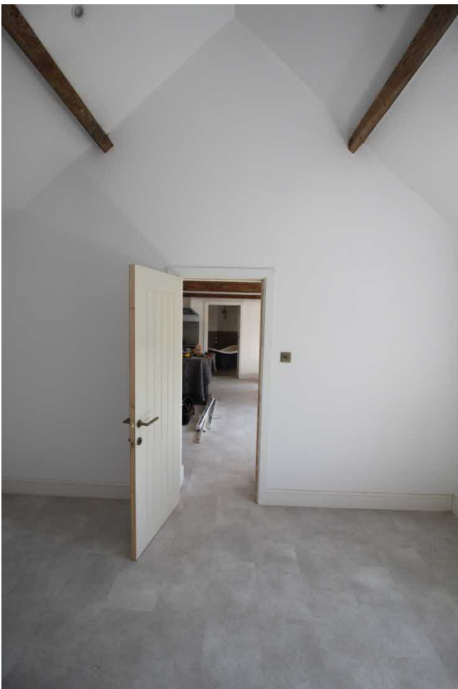
Figure 14 View looking east from inside the first floor, purlin timbers retained.
