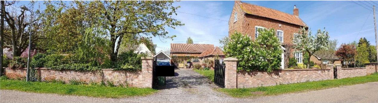
Figure 8 Panoramic view looking west towards the house from Low Road.
