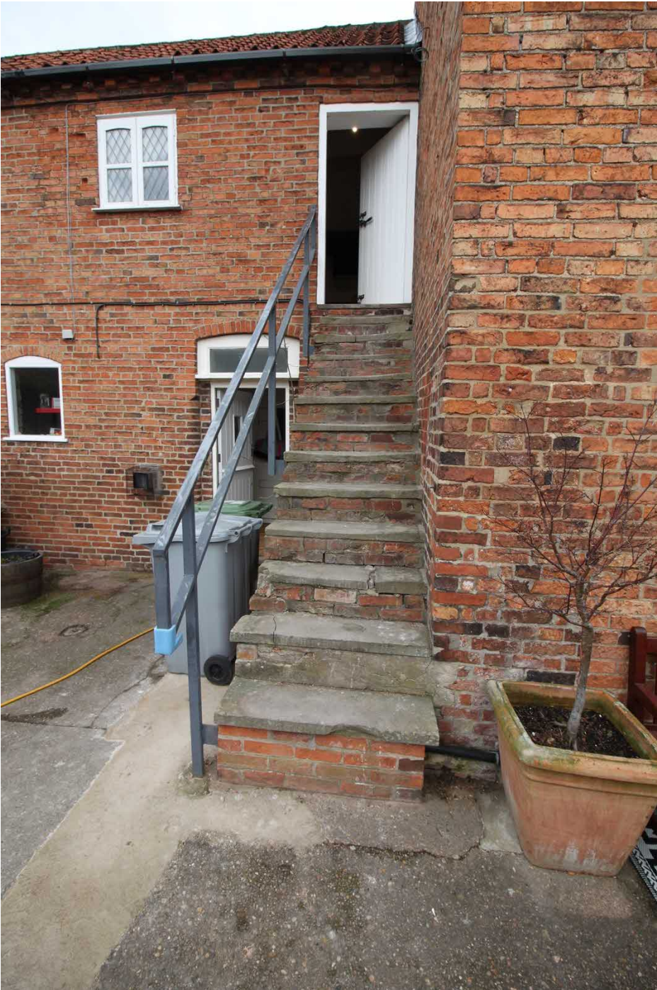
Figure 12 View looking north towards the outbuildings from the rear garden.
