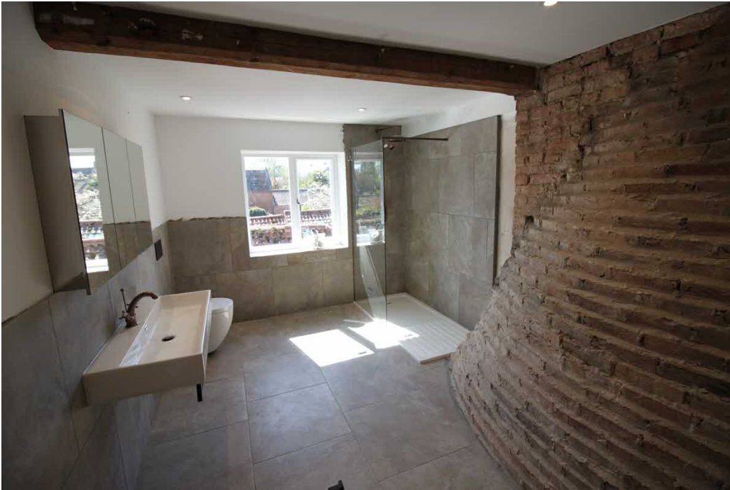
Figure 13 View looking south from inside the first floor, brickwork chimney feature and beam retained.
