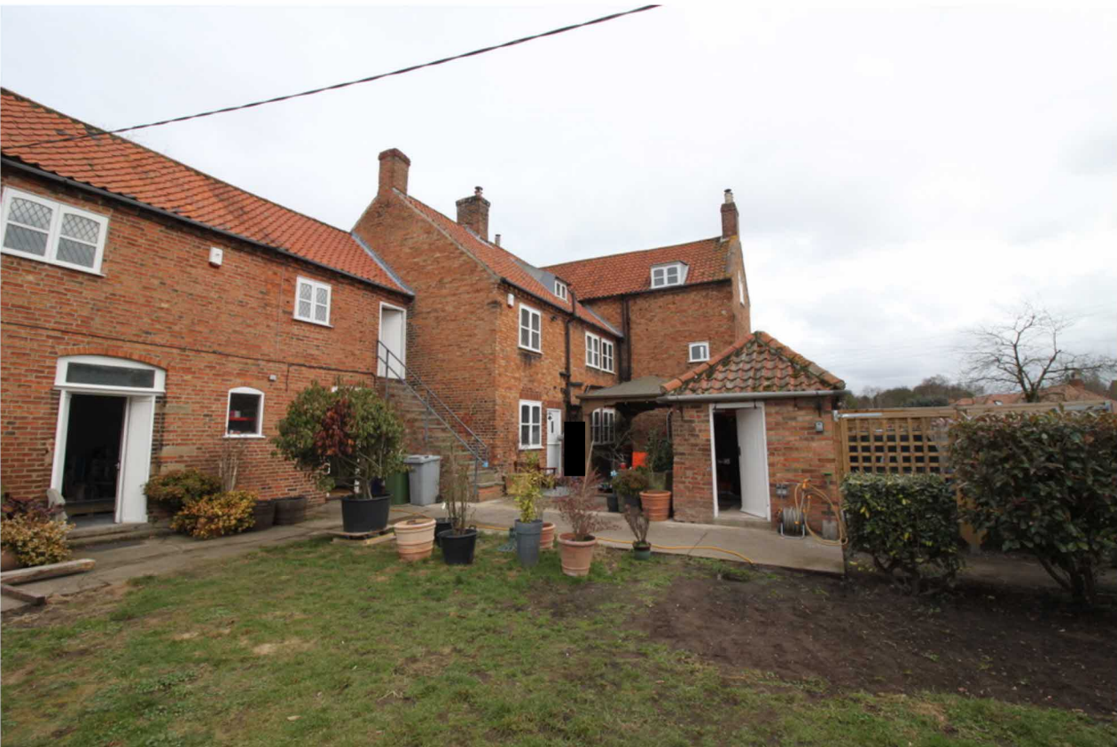
Figure 11 View looking west towards the house from the rear garden.
