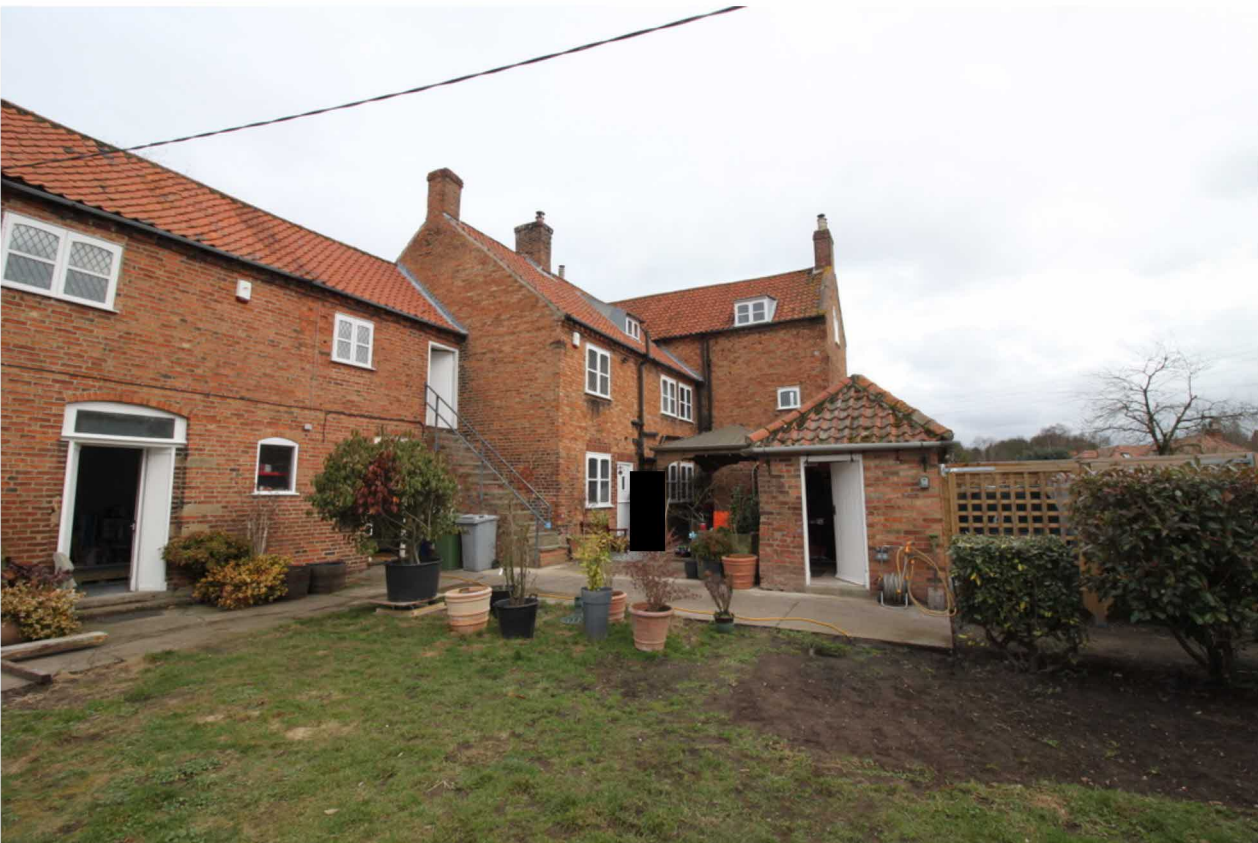
Figure 10 View looking west towards the house from the rear garden.
