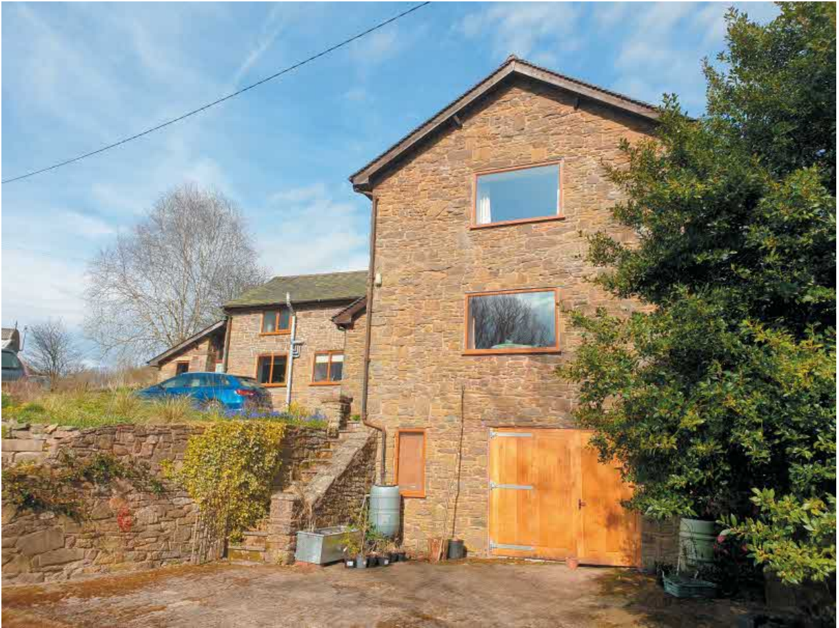
Fig 2, existing house, workshop is behind double doors at lower level
