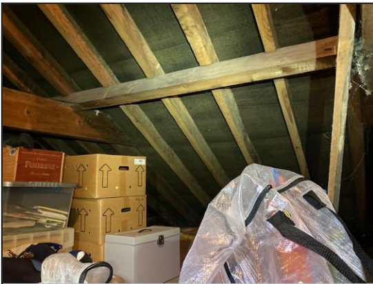
Plate 9: Internal cladding and rafters
