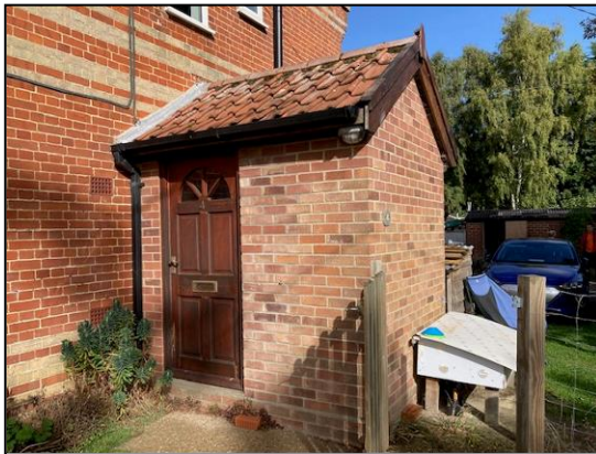
Plate 3: South elevation of the porch
