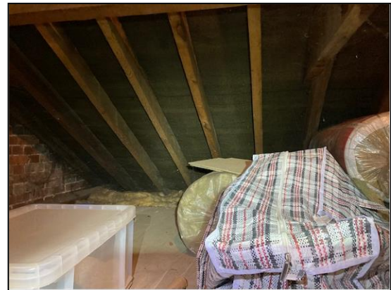
Plate 10: Roof structure at eaves level
