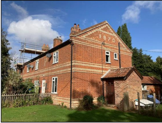
Plate 1: South and east elevations
