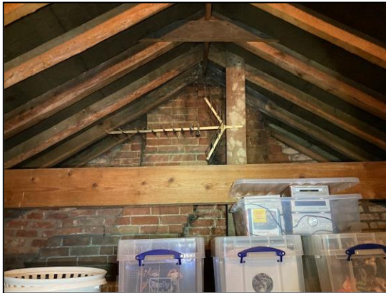
Plate 7: West gable end with chimney
