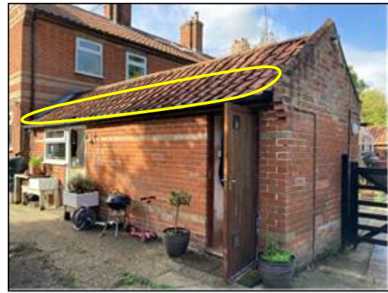
Plate 2: First three rows of pantiles will be lost
