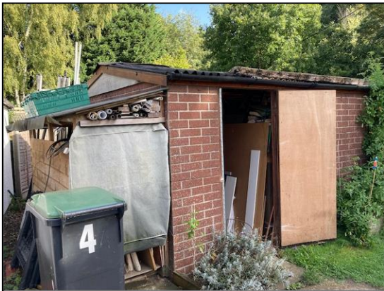
Plate 12: West and south-west corner
