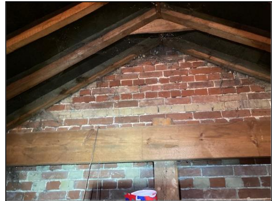
Plate 8: East gable end
