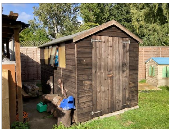
Plate 16: Garden shed, south and east elevations
