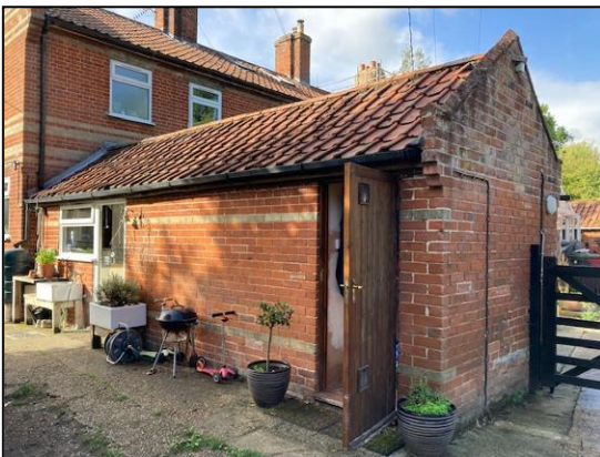
Plate 5: North and east elevations of the extension
