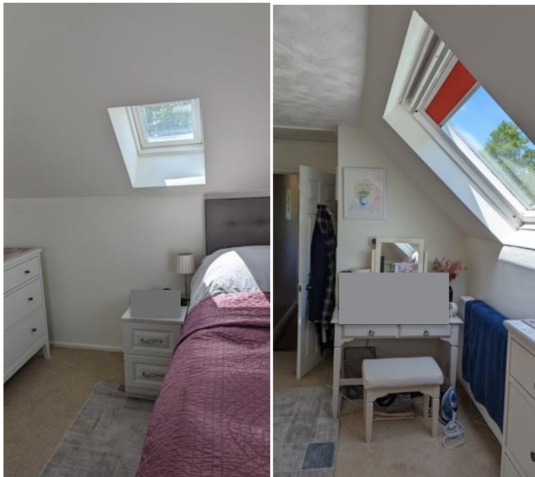
Images 12 & 13: Showing restricted views through roof lights.
