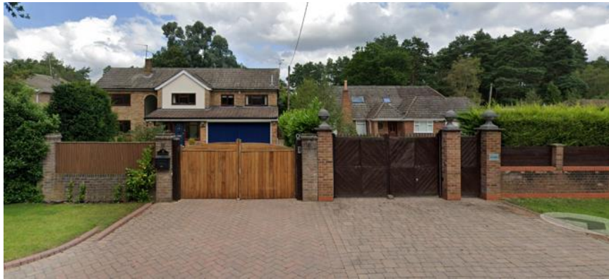
Image 01: Google Maps image showing Teleris and neighbouring two-storey 70s detached.
