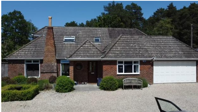
Image 05: Front elevation – photograph of existing property.
