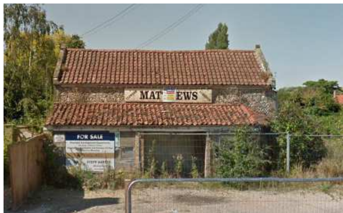
Existing building prior to the commencement of conversion works
