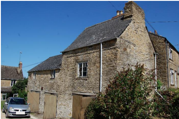
Photograph 1. The south-western (front) and south-eastern elevations of the outbuilding.
