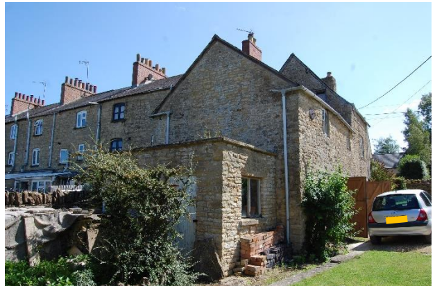
Photograph 2. The north-western elevation of the outbuilding.
