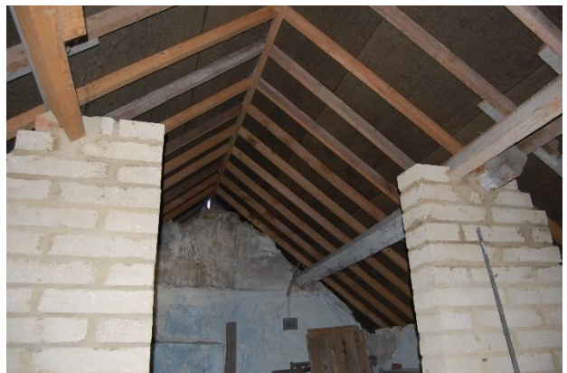
Photograph 6. The central and north-western second floor rooms.
