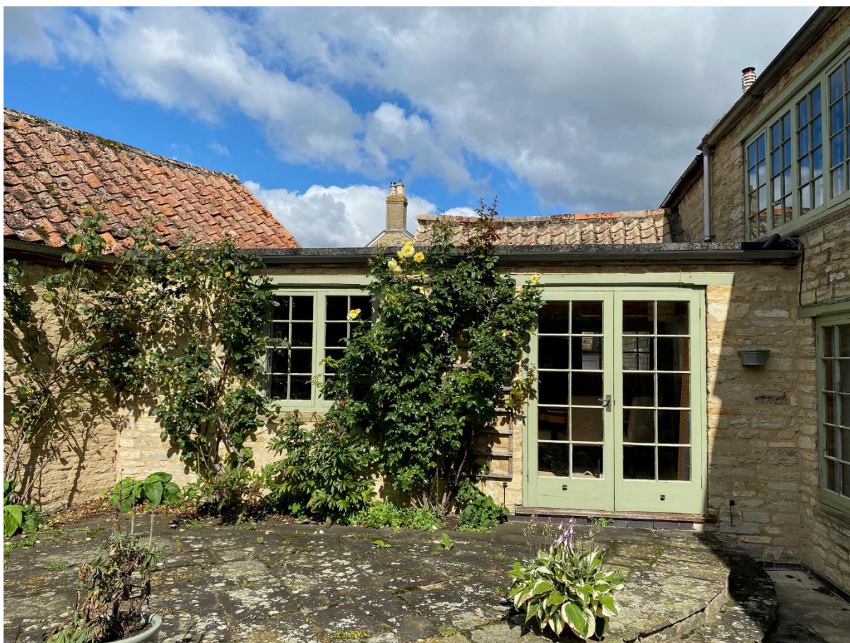
Fig 5 Current link structure to be demolished/rebuilt
