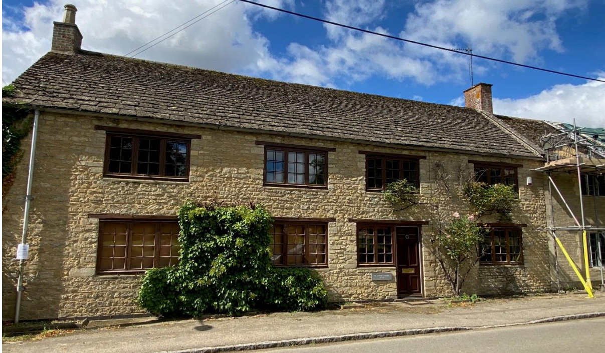
Fig 5 Current dark stained single glazed windows in “newer” cottage to be replaced
