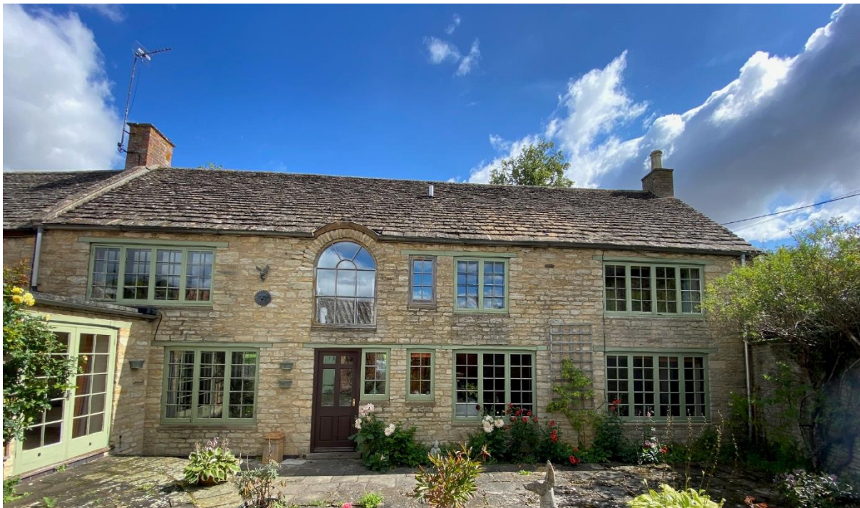
Fig 8 Rear windows of "newer" cottage to be replaced, smaller livingroom window to be adapted to doors to provide direct access into courtyard space
