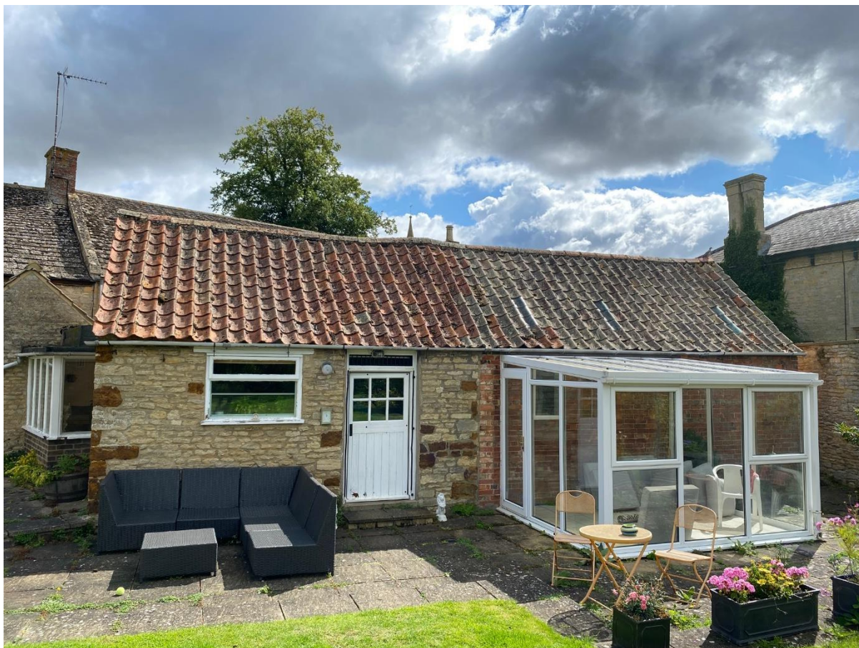
Fig 2 Current rear south wing, conservatory and brick elements to be demolished
