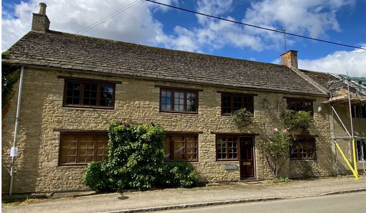
Fig 5 Current dark stained single glazed windows in “newer” cottage to be replaced
