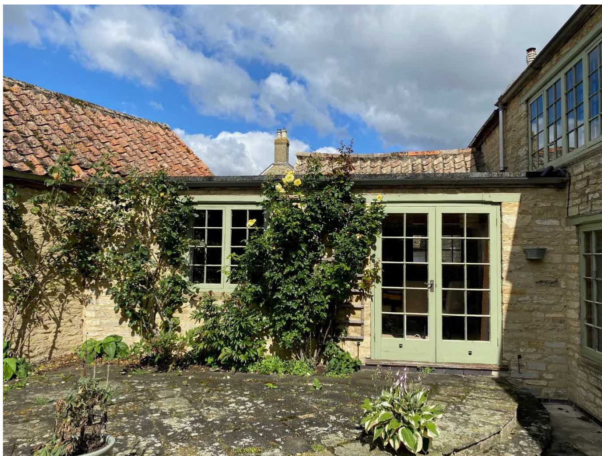
Fig 5 Current link structure to be demolished/rebuilt
