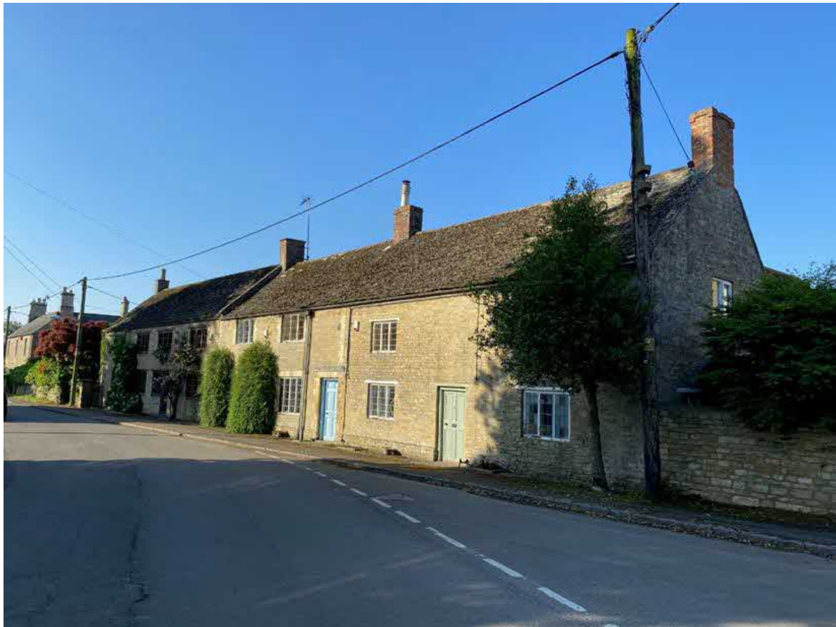
Fig 1 View of property from Min Street, with No 61 in the foreground
