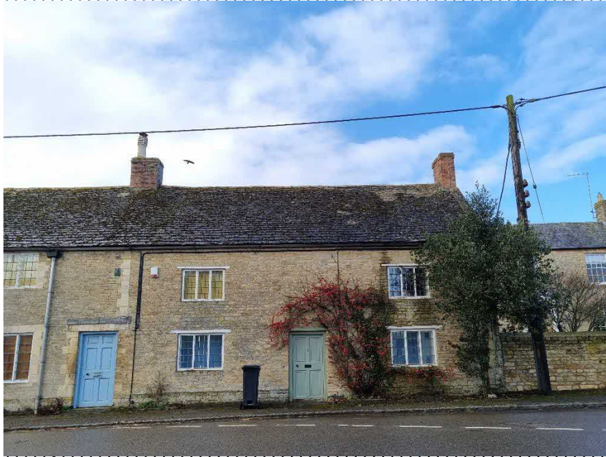
Plate 5. General View of No.61
