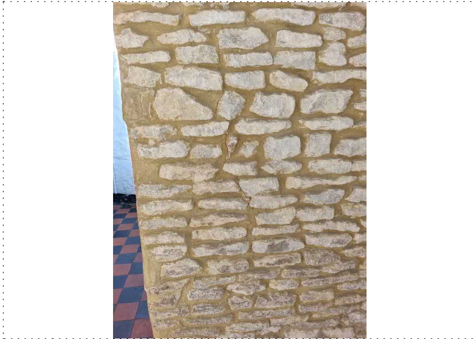
Plate 27. Minor movement within link.
