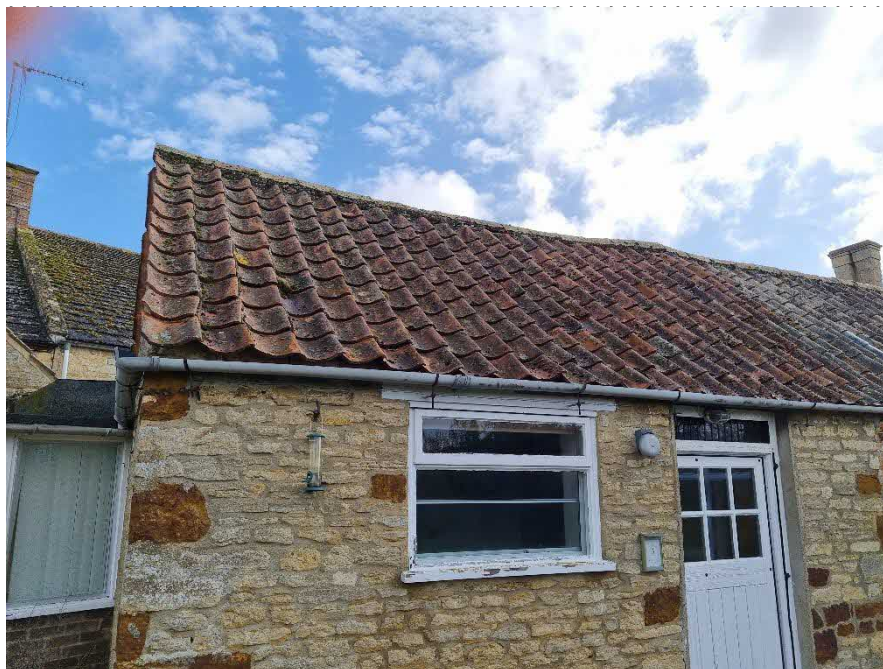
Plate 15. Roof over kitchen (former stable)
