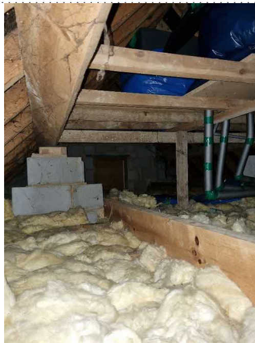
Plate 18. Roof over No. 59
