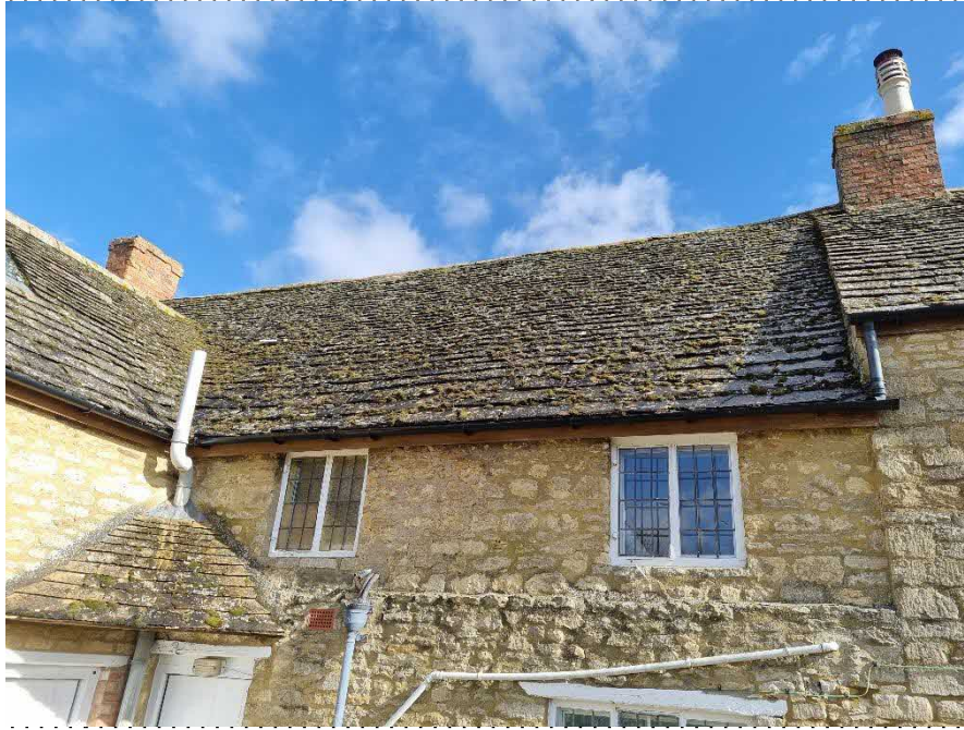
Plate 11. Rear elevation of No. 61
