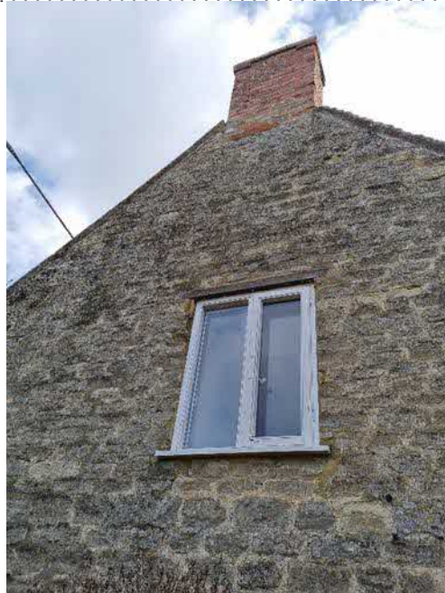
Plate 7. Typical condition of North gable.
