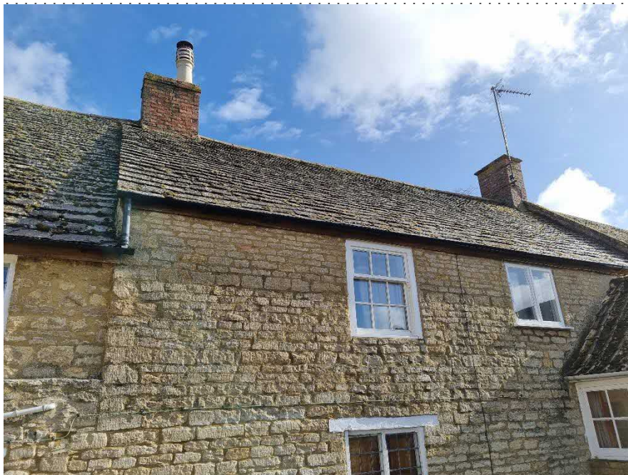
Plate 12. Rear elevation of No. 59
