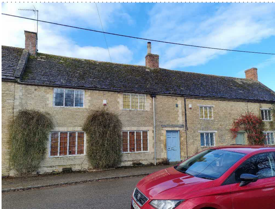
Plate 4. General View of No.59
