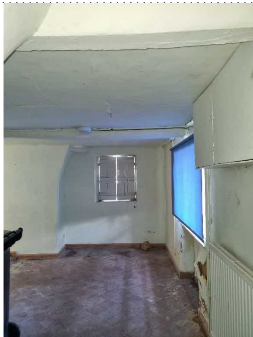
Plate 24. Typical view in No.61 Ground floor.
