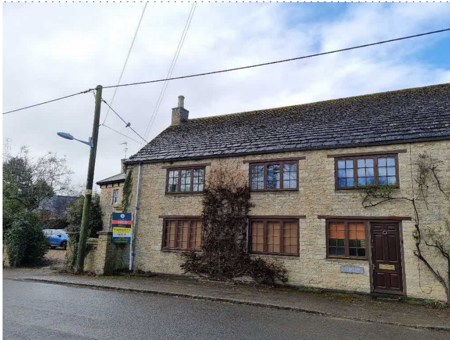
Plate 2. Roof over No.57
