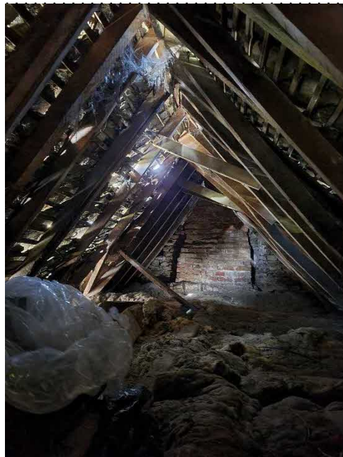
Plate 20. Roof space over No. 61.
