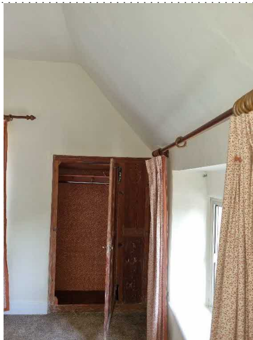
Plate 22. Typical view of No.61 1st floor finishes.
