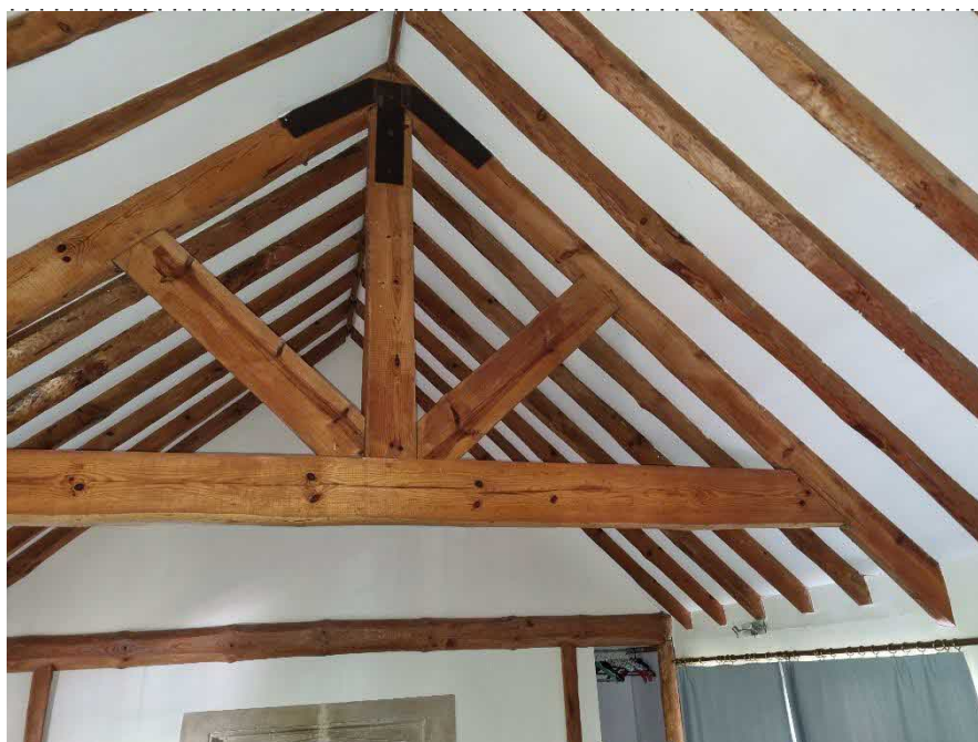
Plate 16. Roof over No.57
