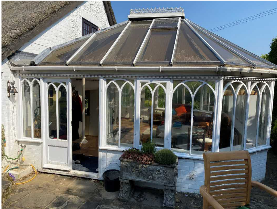
Figure 5. Conservatory looking north
