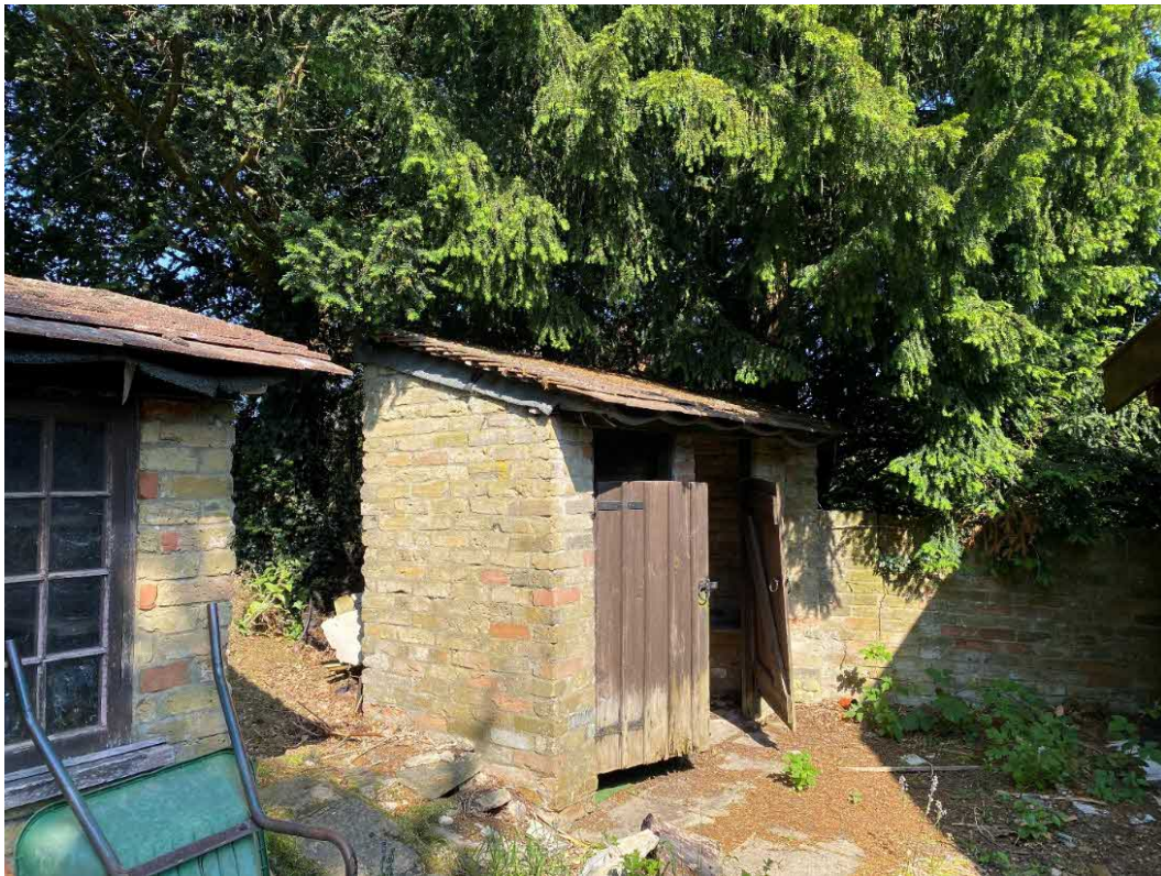
Figure 9. Sheds looking north
