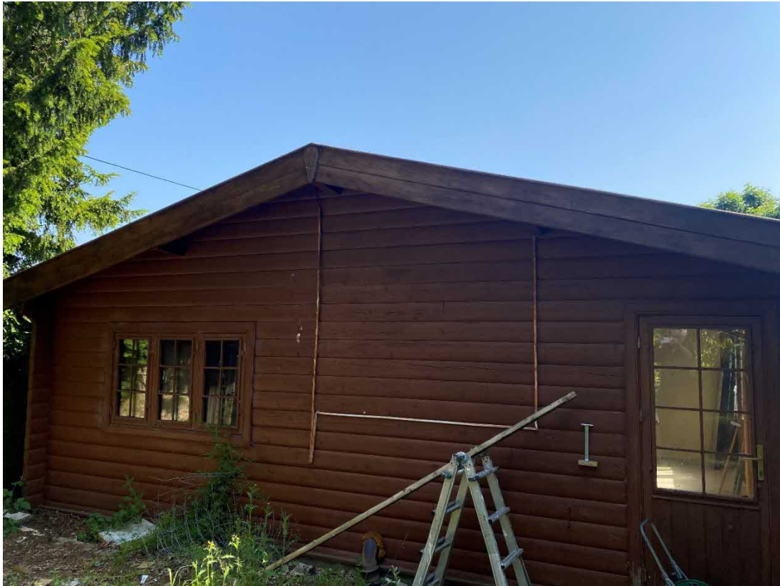
Figure 7. West gable of garage looking northeast
