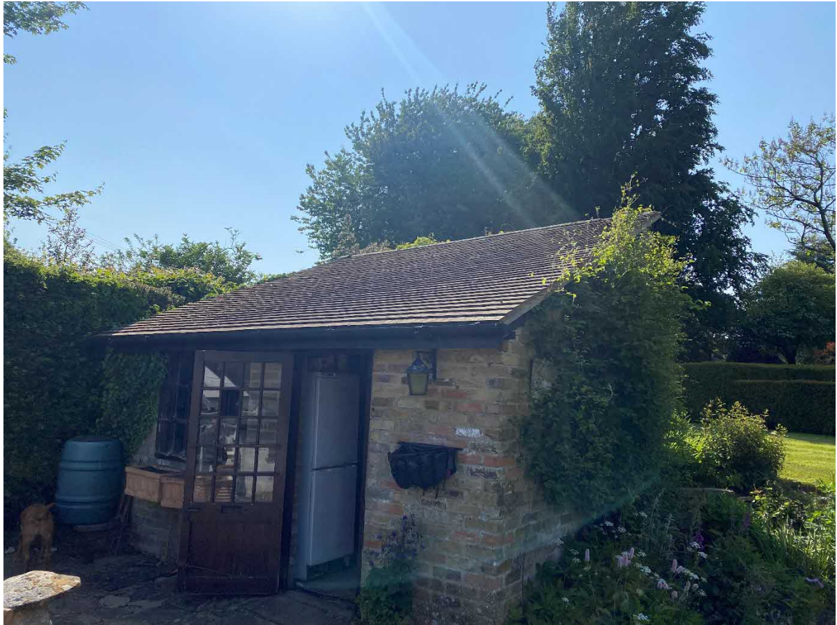
Figure 6. Utility building looking southeast.
