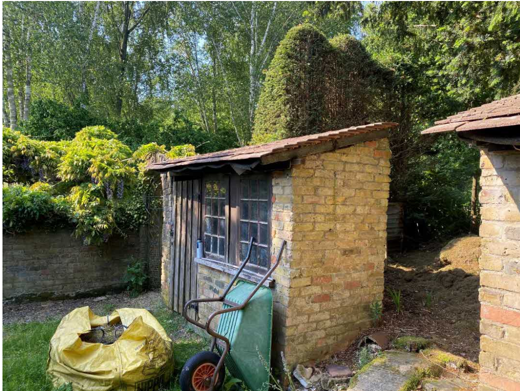
Figure 10. Sheds looking south
