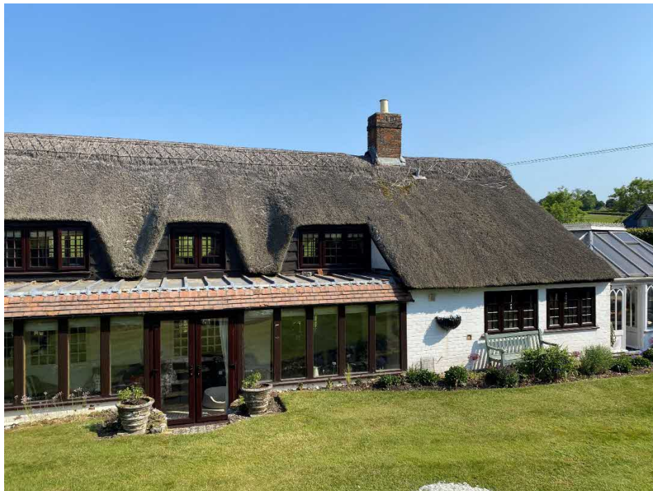
Figure 4. Southern elevations looking north.
