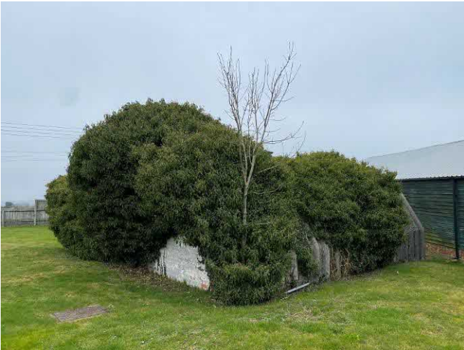
South and east elevations of Building 3
