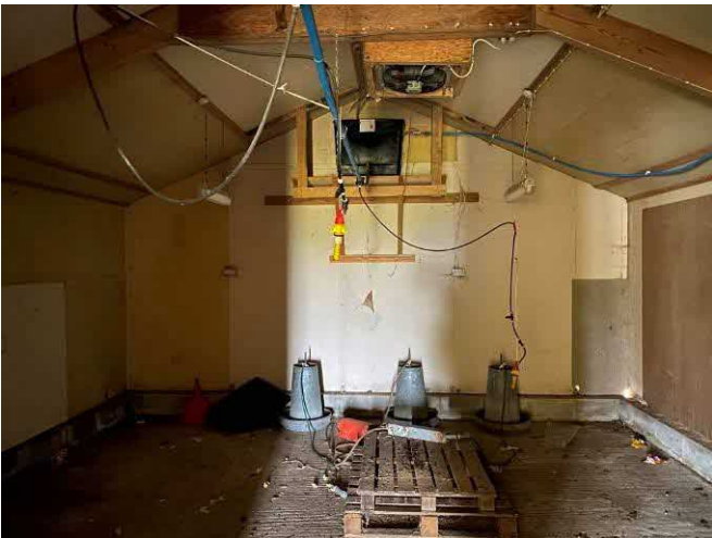
East room of Building 5
