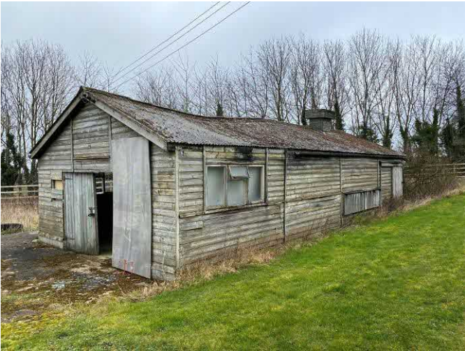
South and west elevations of Building 5
