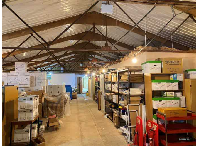
Interior of warehouse in southeast half of Building 2
