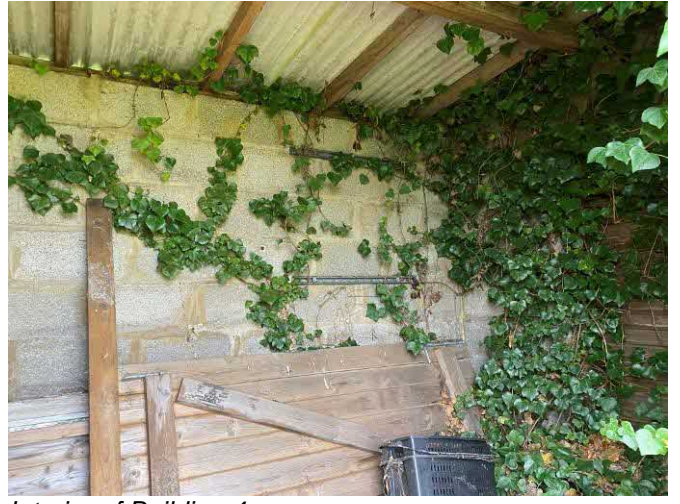
Interior of Building 4
