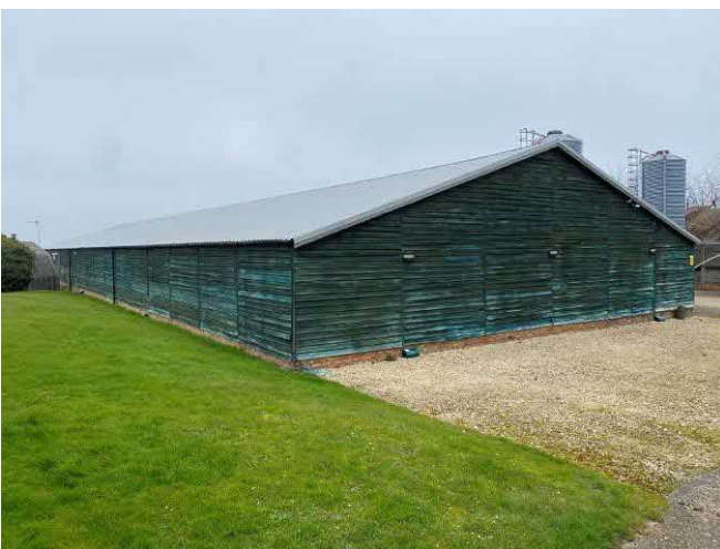
Southwest and southeast elevations of Building 2
