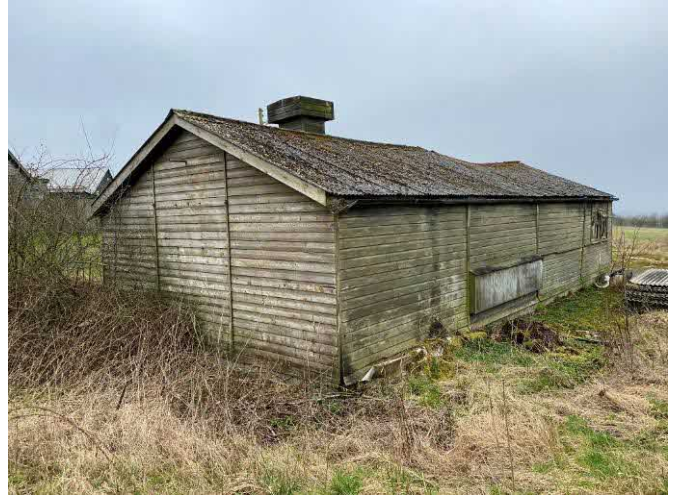
North and east elevations of Building 5
