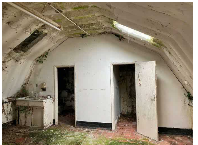
Enclosed rooms at south end of Building 3
