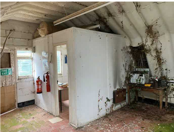
Enclosed office at north end of Building 3
