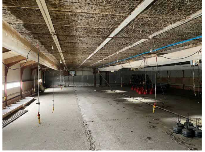
Interior of Building 1
