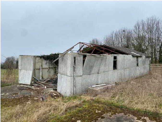
South and east elevations of Building 6
