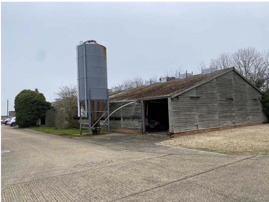
Southeast and southwest elevations of Building 1
