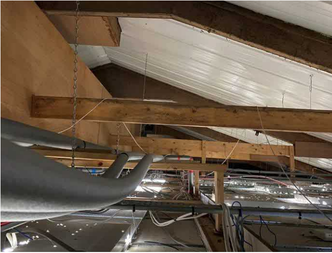
Roof space above offices in Building 2
