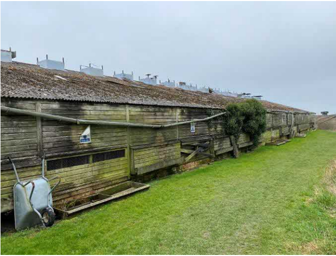
Northeast elevation of Building 1
