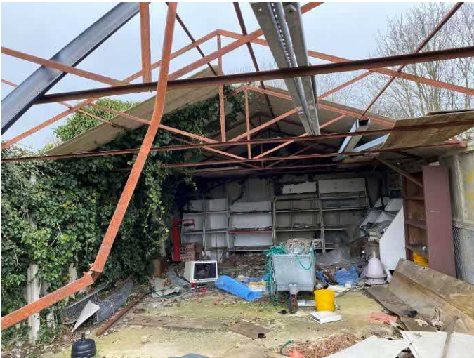
Interior of Building 6
