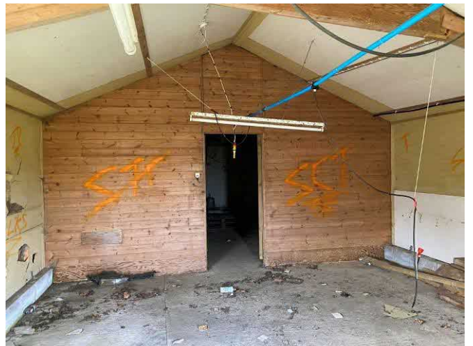
West room of Building 5
