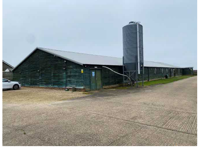
Southeast and northeast elevations of Building 2
