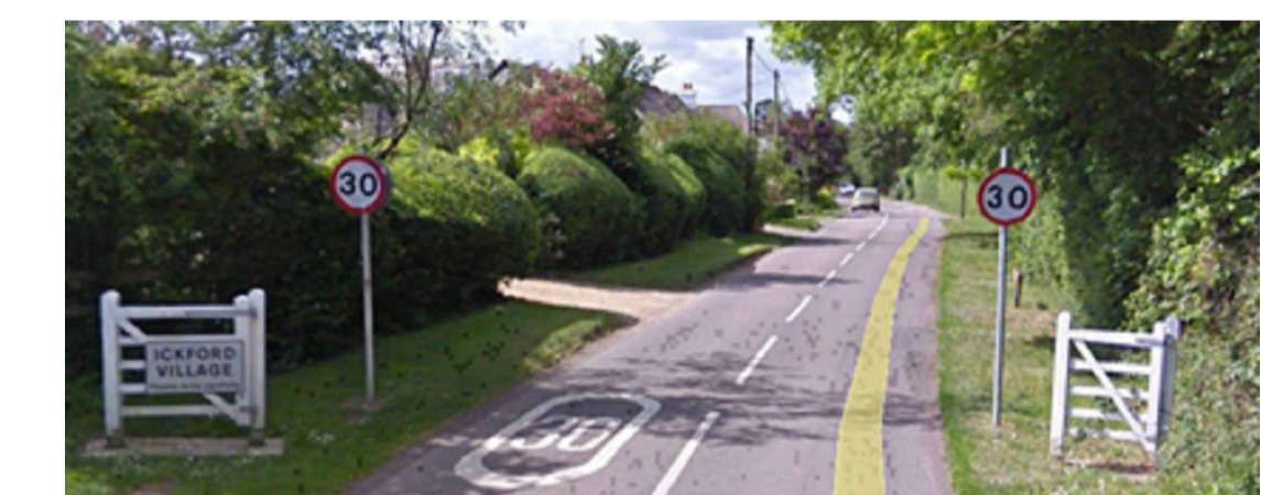
Existing speed limit signs to remain in place with additional gateway feature added including 30mph roundel marking and red band surfacing.
