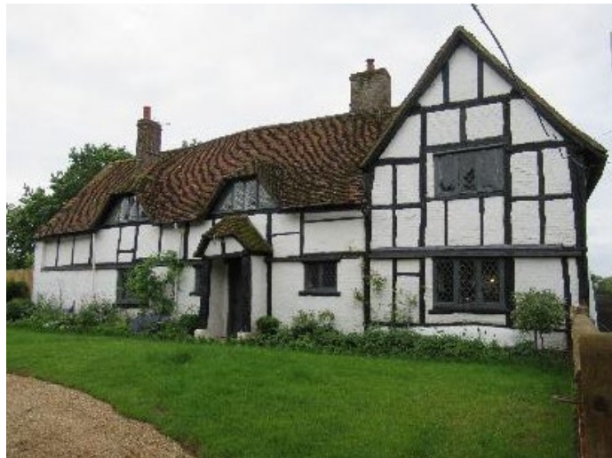
Front elevation of the Old Manor
