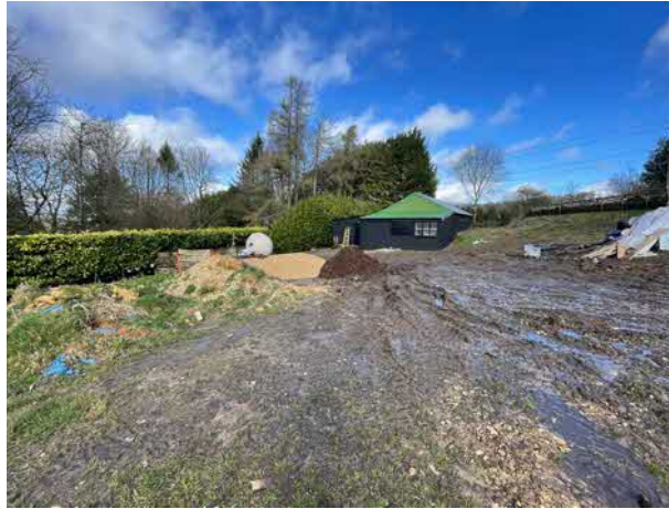
Photograph 4: Area of bare ground to the south of the building.
