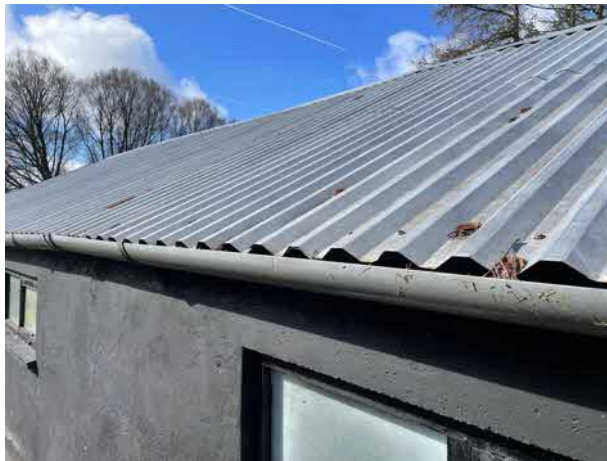
Photograph 19: Gaps along the bottom of Section B corrugated roof.
