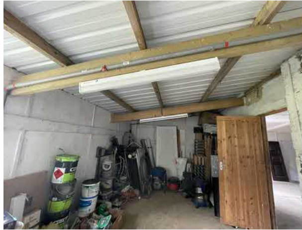
Photograph 18a: Section A interior in 2023.
