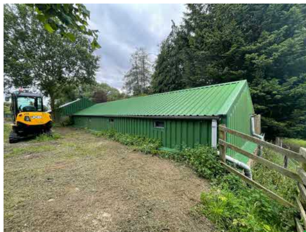
Photograph 15a: East elevation of Section D in 2023.
