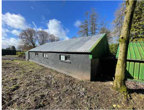
Photograph 14: East elevation of Section B.
