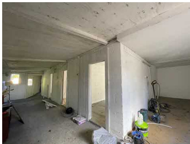
Photograph 20: View of Section B interior with inaccessible roof void above.
