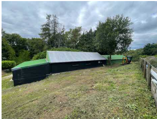
Photograph 1a: General view of the building on site in 2023.
