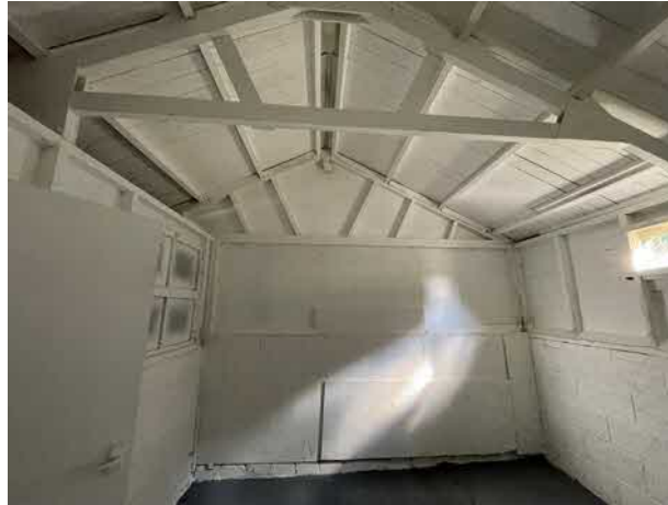
Photograph 24 : Section D interior with timber sarking boards lining the roof.
