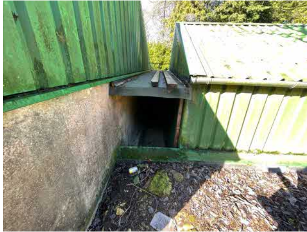
Photograph 16: Porch area between Sections B and D.
