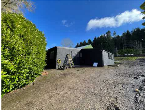
Photograph 12: View of the southwest corner of the building with Section C attached to the west elevation.
