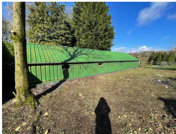
Photograph 15: East elevation of Section D.
