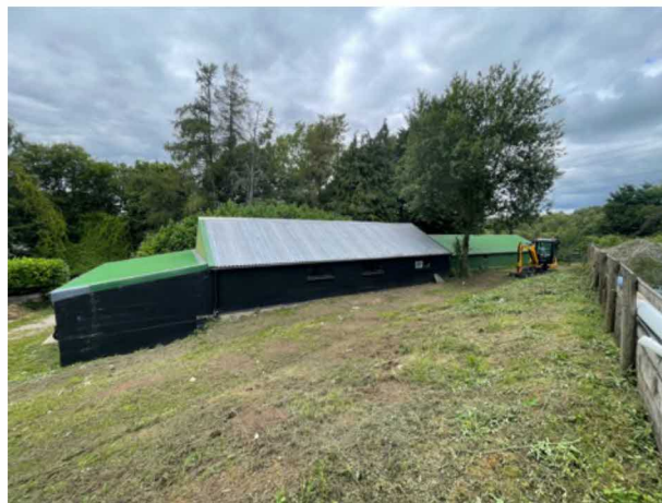
Photograph 11a: View of Building in 2023.
