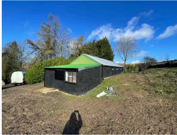
Photograph 1: General view of the building on site.
