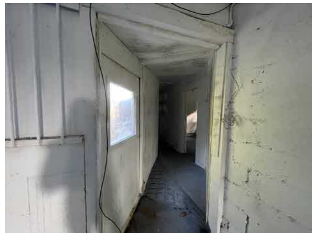
Photograph 22: Section E walkway interior joining Sections C and D.
