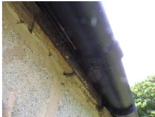
Fig. 9 Tightly fitting fascia board
