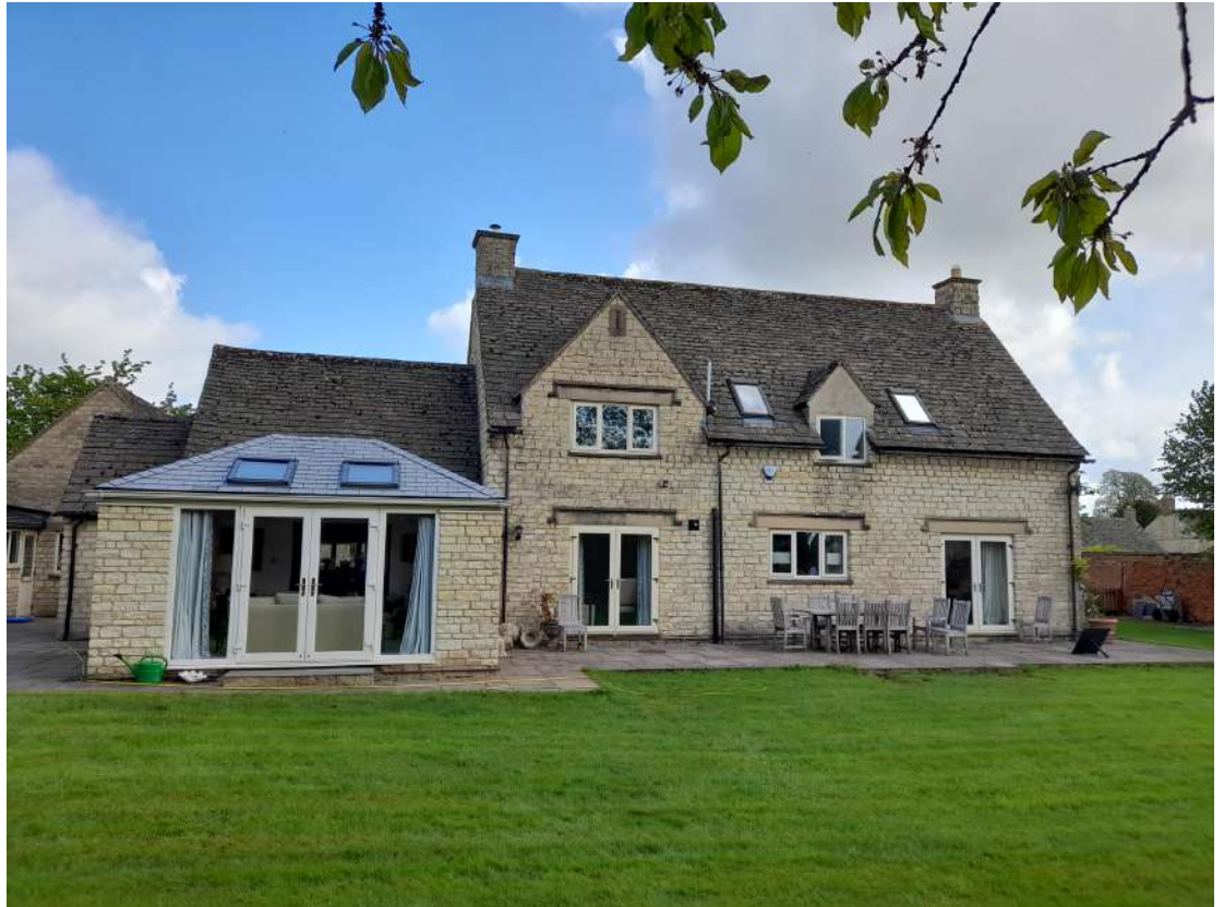
Above: Rear elevation, garden room with synthetic slates
