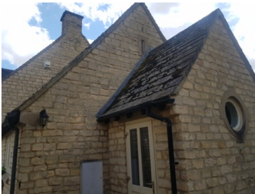
Photo 9: B2 - West facing elevations
