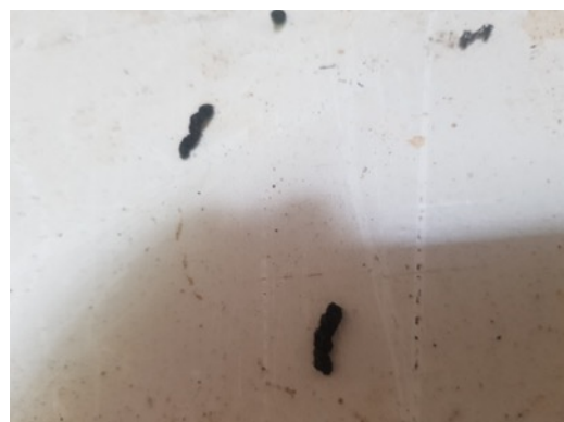
Photo 6: B1 - Scattered bat droppings on floor of loft
