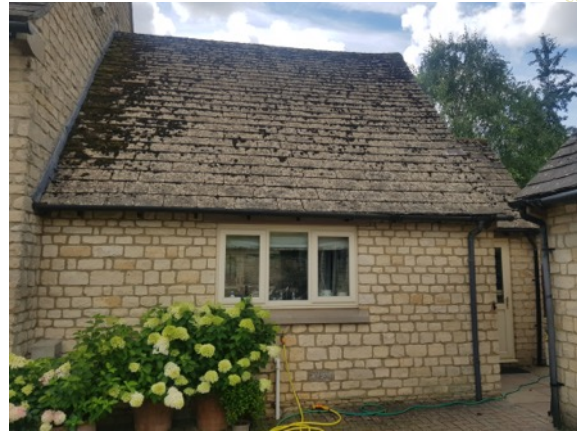
Photo 8: B2 - North facing elevation
