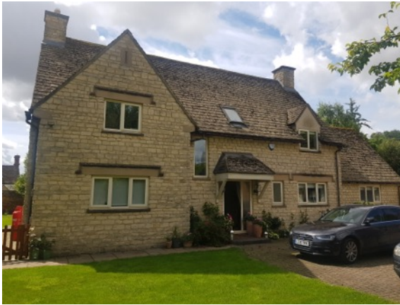
Photo 1: B1 - North facing elevation
