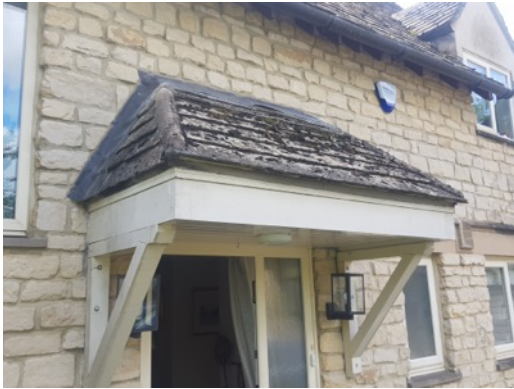
Photo 3: B1 - Porch to be removed and replaced
