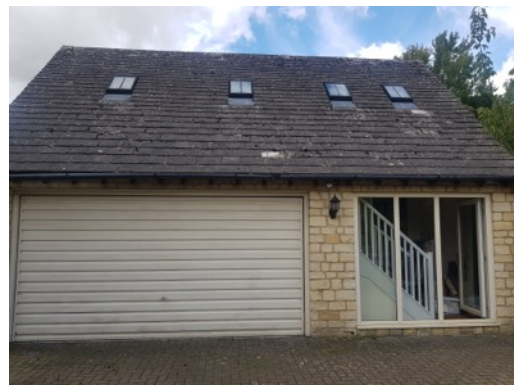
Photo 12: B3 - East facing elevation
