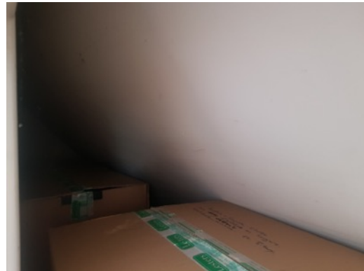
Photo 16: B3 - Boarded out eaves roof spaces
