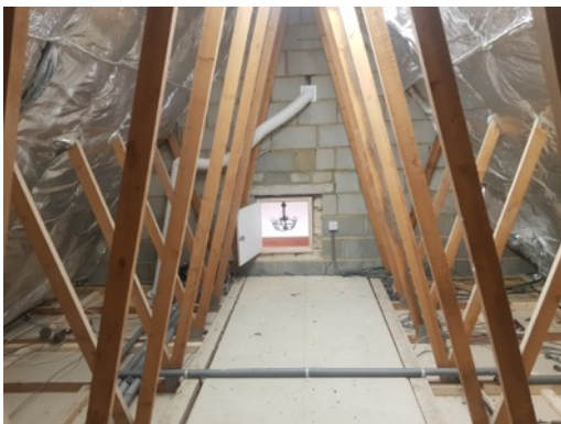
Photo 11: B2 - Interior view of loft void
