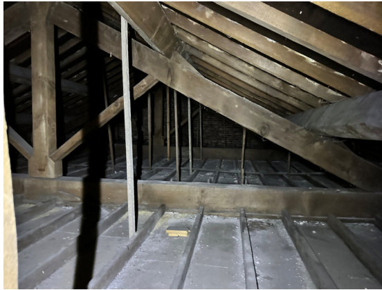
View of existing roof space.
