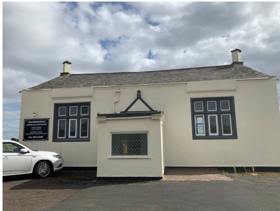
View of front elevation with central porch to be removed.
