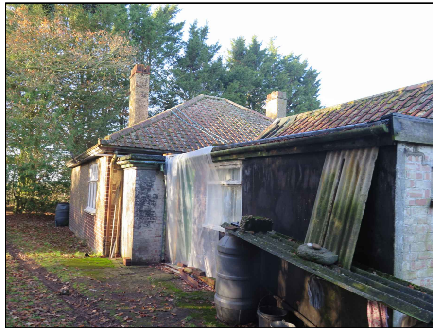
South Elevation of existing dwelling
