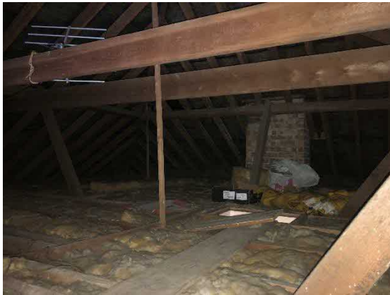
Figure 7: Hipped roof loft space looking north
