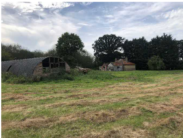
Figure 9: Nissan hut looking south-west
