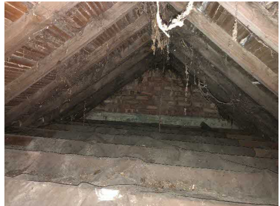
Figure 8: Loft space looking west
