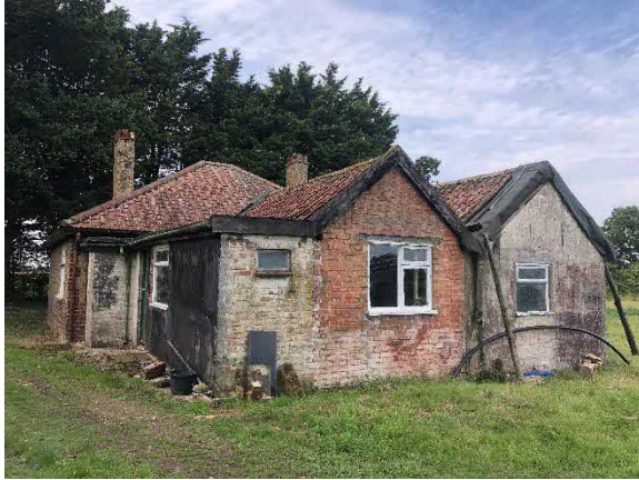
Figure 5: Building looking north-west
