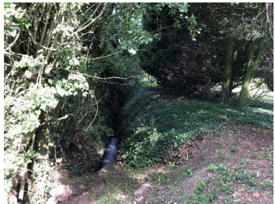
Figure 2: Western boundary ditch looking north
