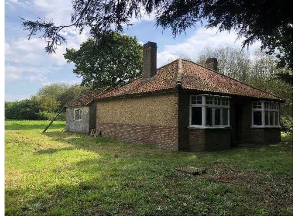
Figure 6: Building looking south-east
