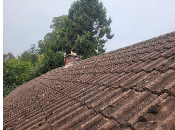
P4: Example of the tight-fitting roof and ridge-tiles
