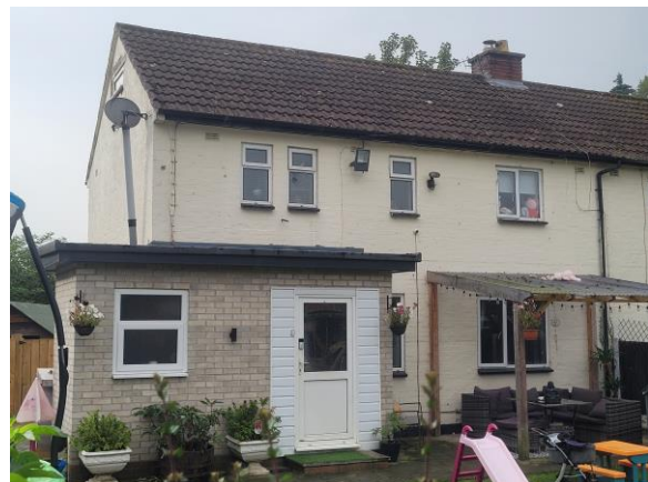
P2: NE (gable) + NW (front) elevations: looking SW
