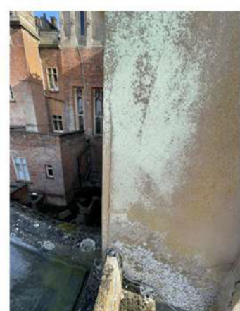
15- Vertical split of render at return to rear elevation
