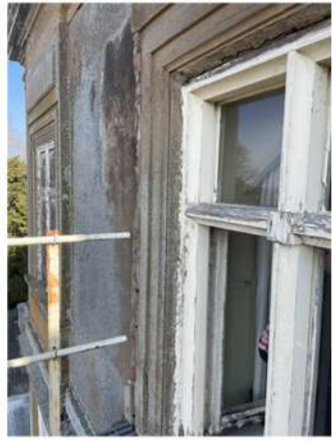
5- Defective, moulded string course pulling away
