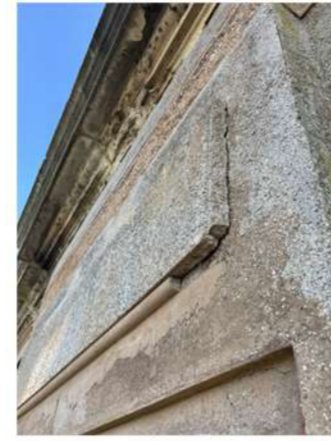
7- Debonded render panel & loss of roll mould
