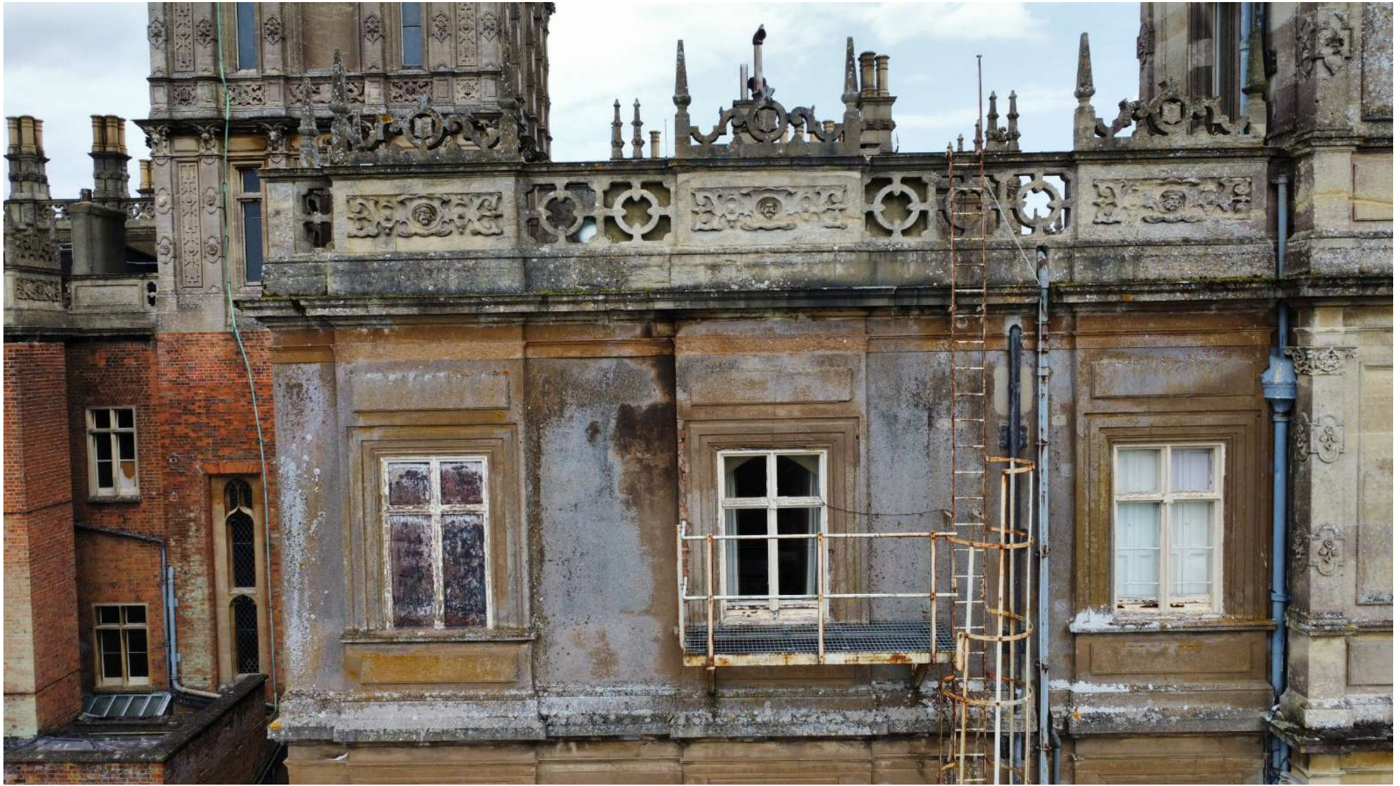
Fig. 6 (below) A drone captured view of the site. Note the dummy window to the left hand side.
