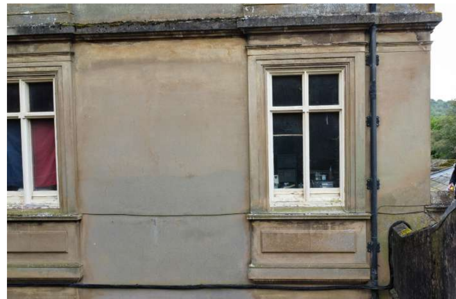
Fig. 36 The adjacent North facing facade in better condition.
