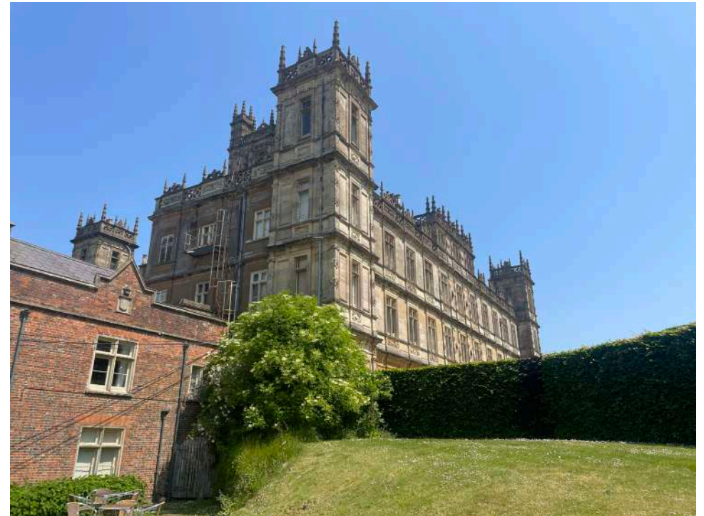
Fig. 3 (below) Highclere Castle's rendered West Front and stonework South Front and towers, viewed from the southwest (BHB Architects 2023)
