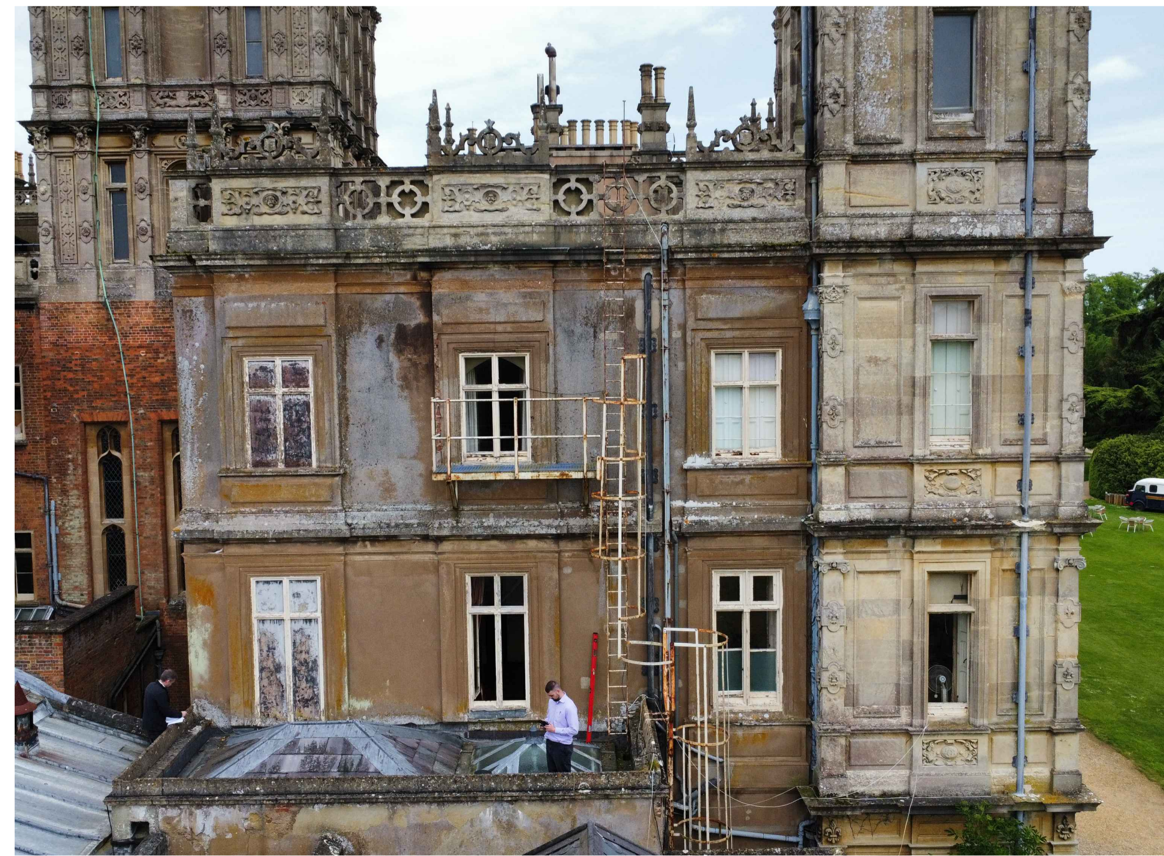
Fig.1 - West Wing Elevation - General Photo Not to Scale
