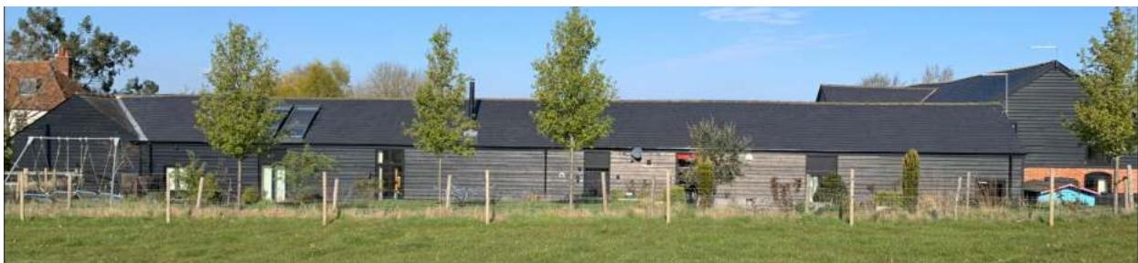
Photo of large roof-lights in situ
