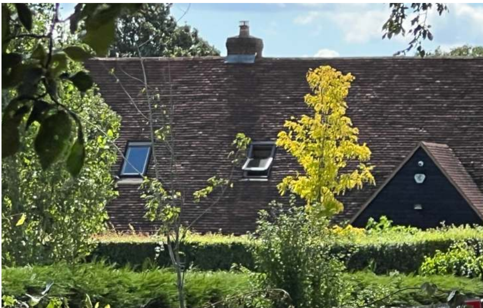
Conservation-style roof-lights on the neighbouring Grade II listed Great Barn, as viewed from the public footpath to the NW. The proposed roof-lights will have a comparable form, profile and visual impact, albeit with considerably reduced public visibility
