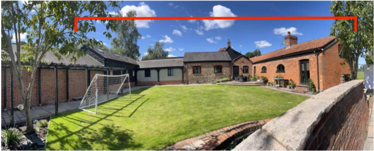
Site photograph demonstrating the extent of the building's various roofs & the very small total % of roofs to be covered by roof-lights
