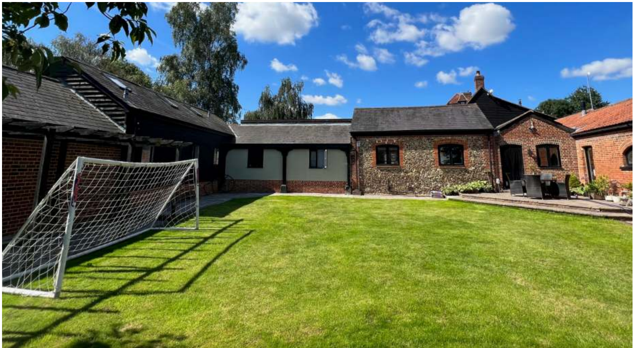
The site's private, internal courtyard comprises the external part of the site with the most obviously domesticated character
