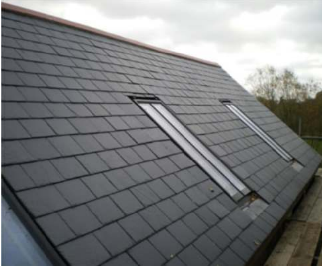
Example of conservation-style roof-lights, sitting flush with the slate roof
