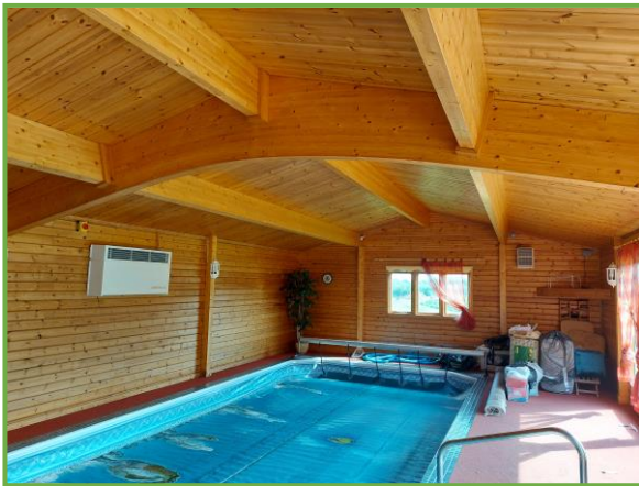
Photo 4: Internal view of B2
