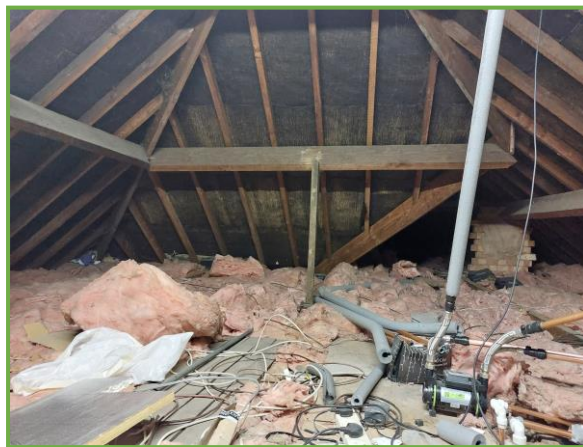
Photo 2: View showing roof void and underfelt.
