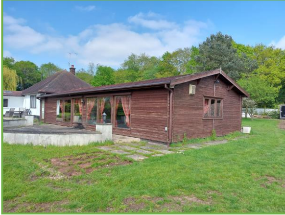
Photo 3: View of timber constructed swimming pool building (B2).
