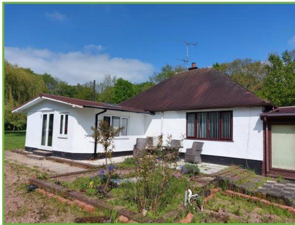
Photo 1: View of Five Acre bungalow with single-storey extension.
