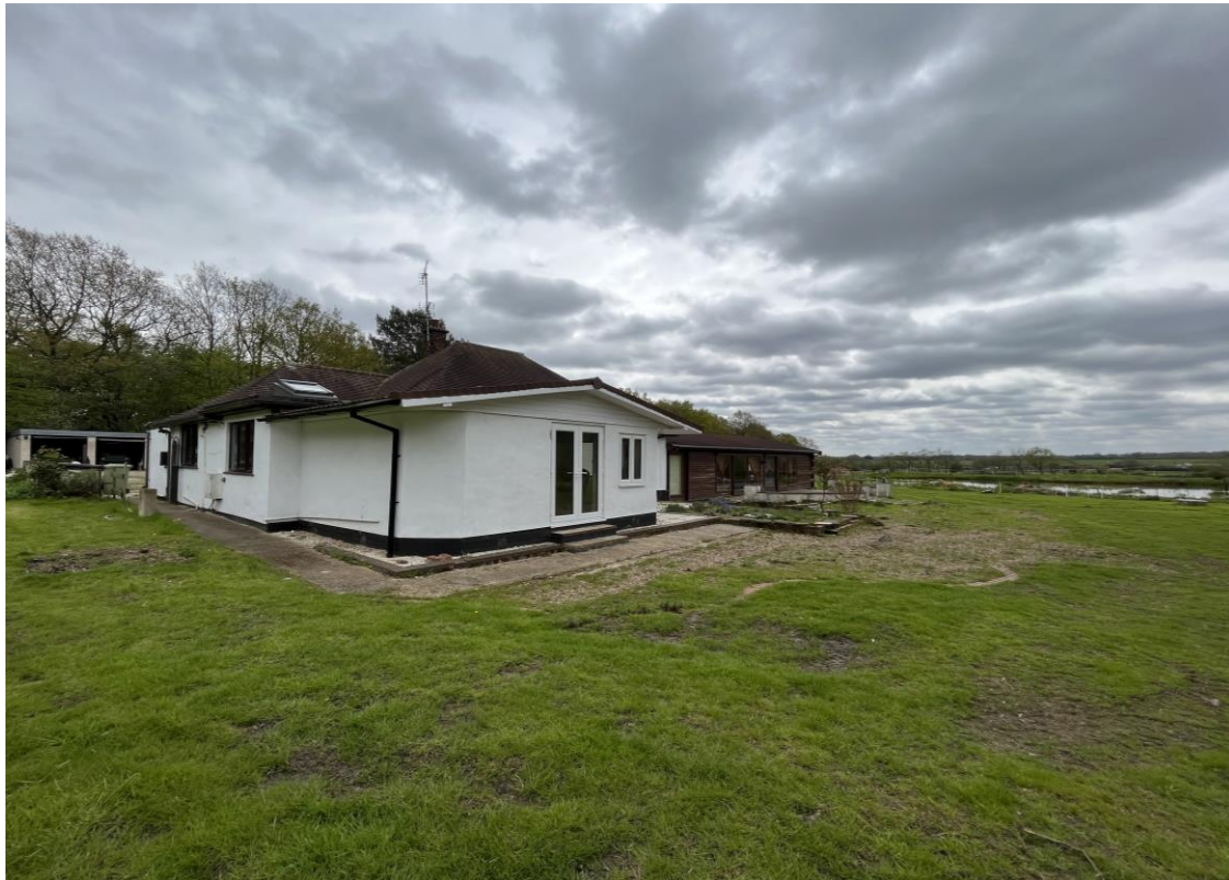
Site for new Dwelling Adjacent Existing Dwelling (To be demolished)
