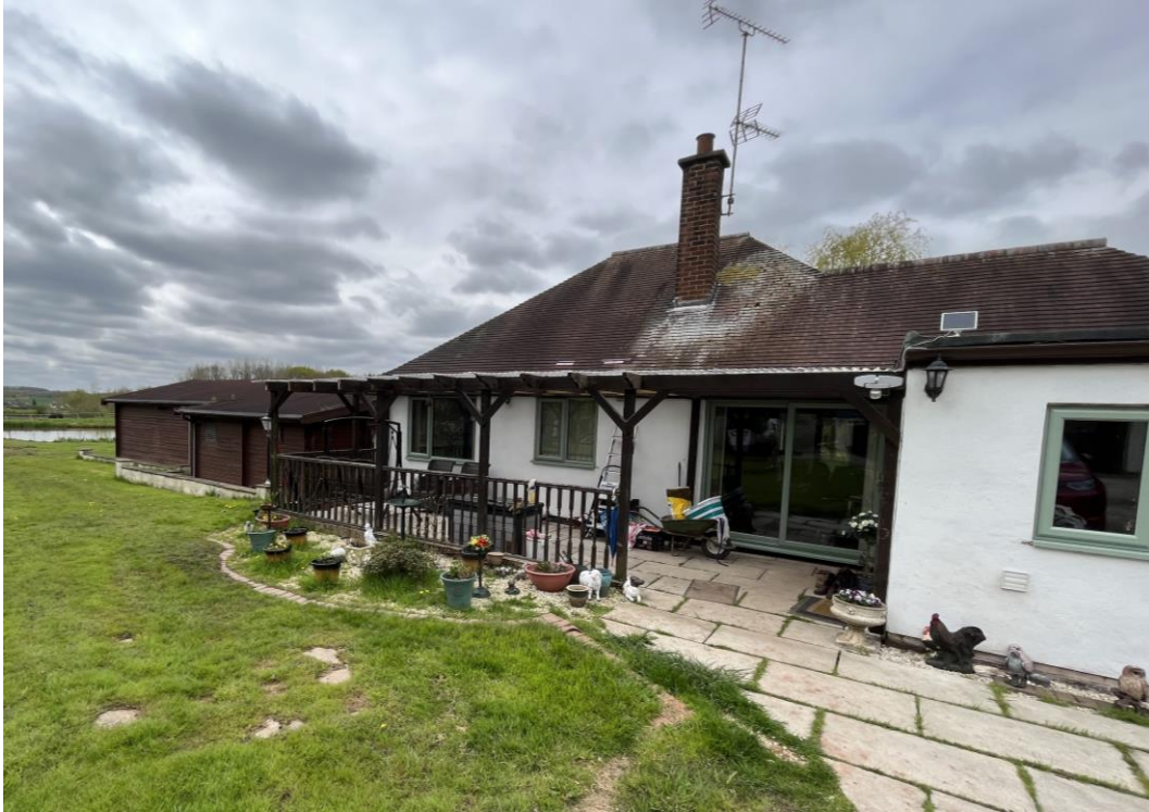
Existing Dwelling Side (East)
