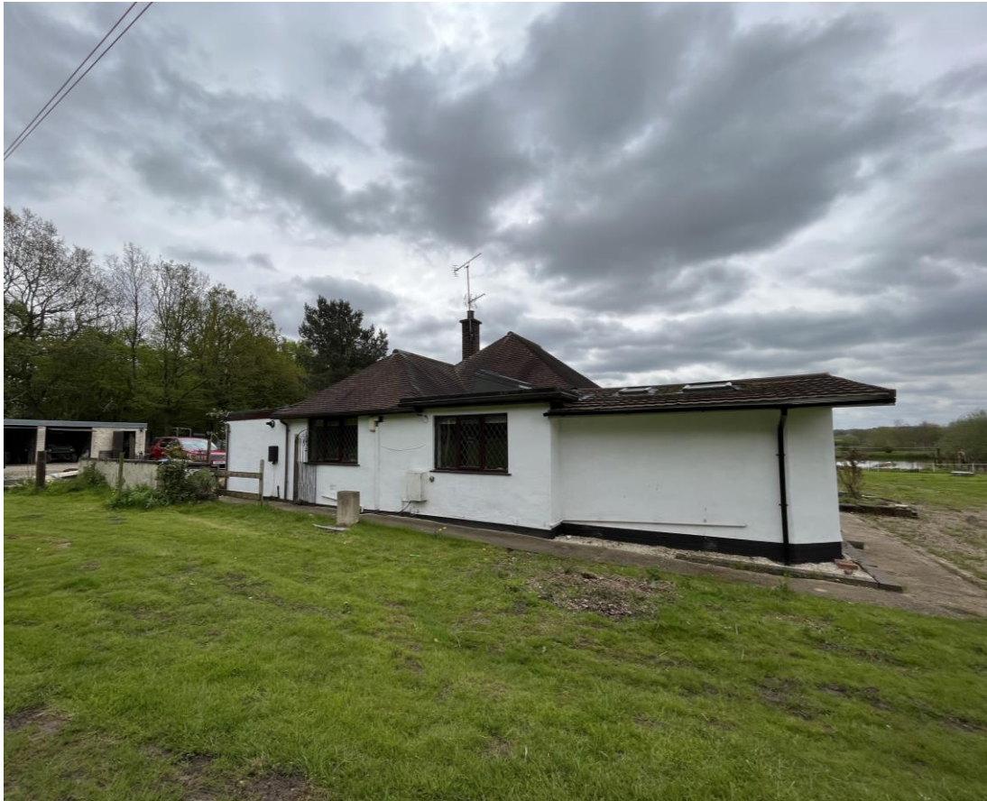
Existing Dwelling Front Elevation (North)
