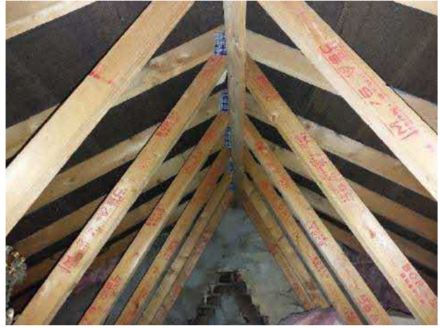
Figure 2. Eastern Roof void of B1
