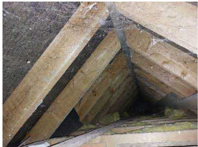
Figure 4. Roof void of B2
