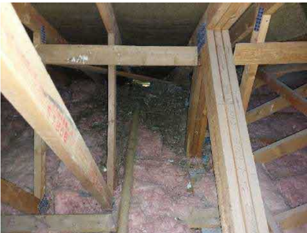
Figure 3. Western roof void of B1 showing old pigeon nest
