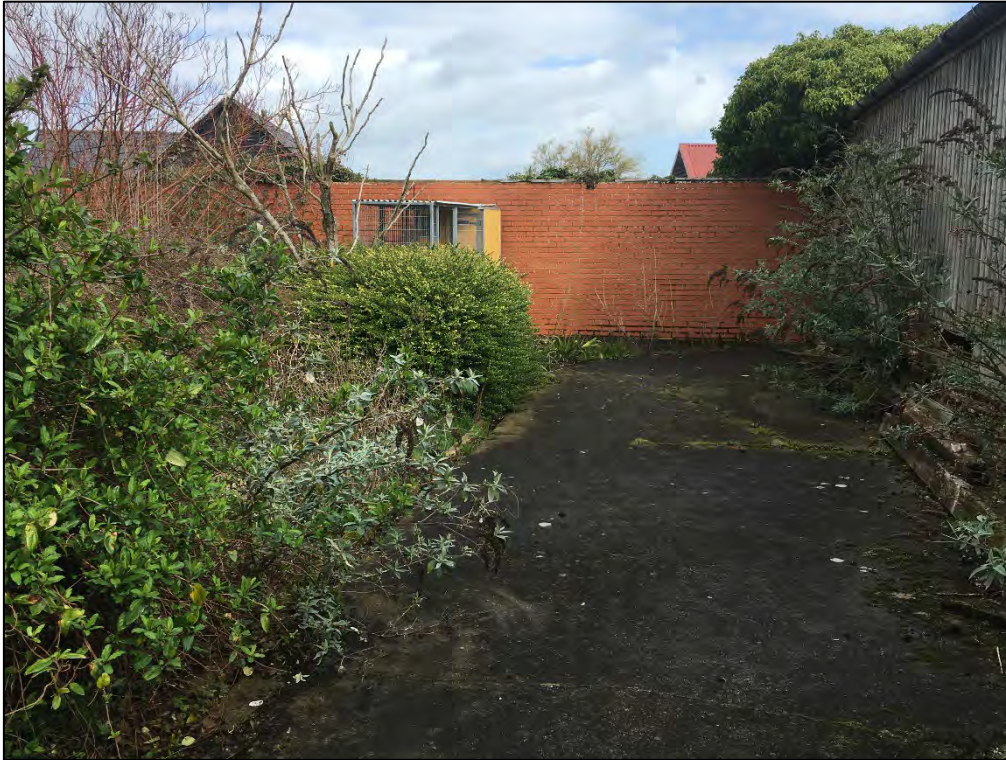
Photograph 23: The courtyard (No 2), with Building 1 on the right.
