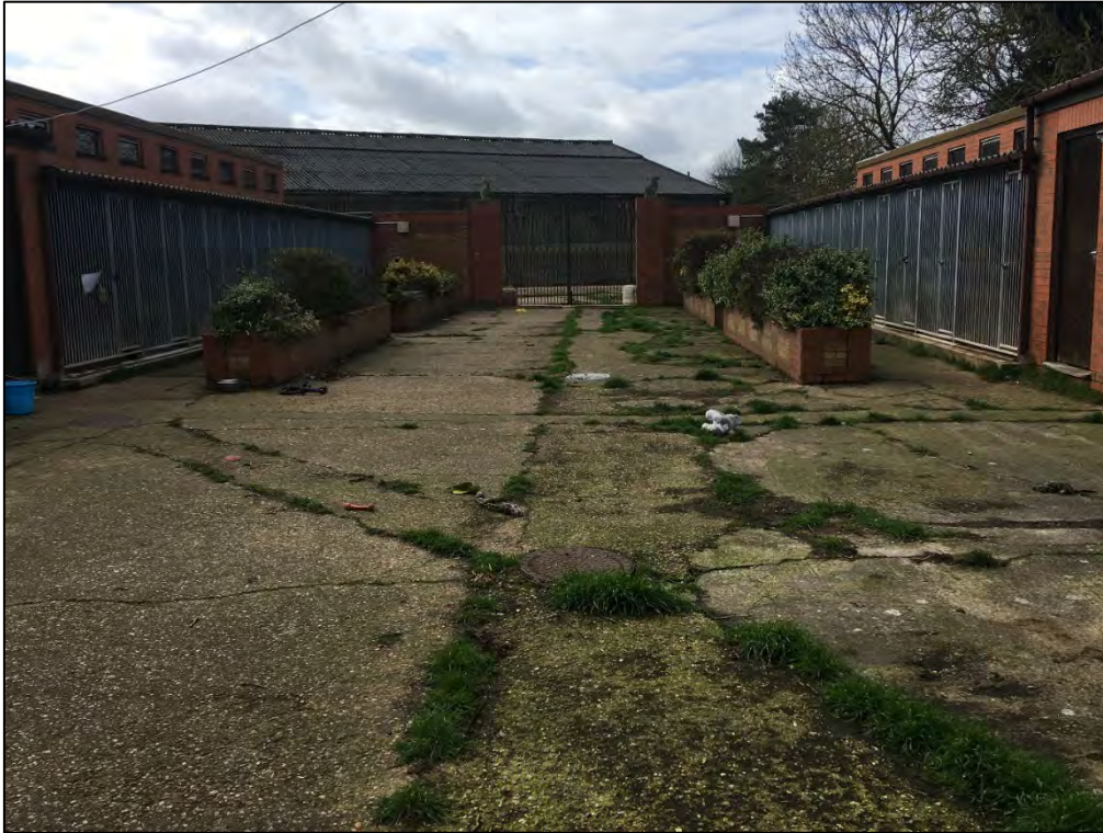
Photograph 13: The main kennel area (Buildings 6 and 7)
