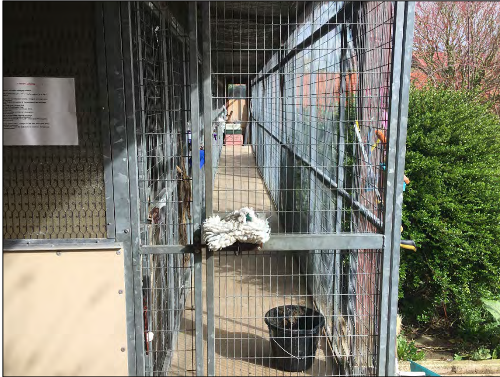
Photograph 19: The cattery, which lies to the rear of Building 3 and is adjoined by an alley to Building 7 (Building 7a).
