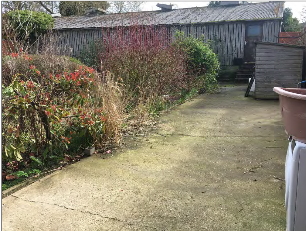
Photograph 20: The courtyard (No 2), between Buildings 7 and 1.
