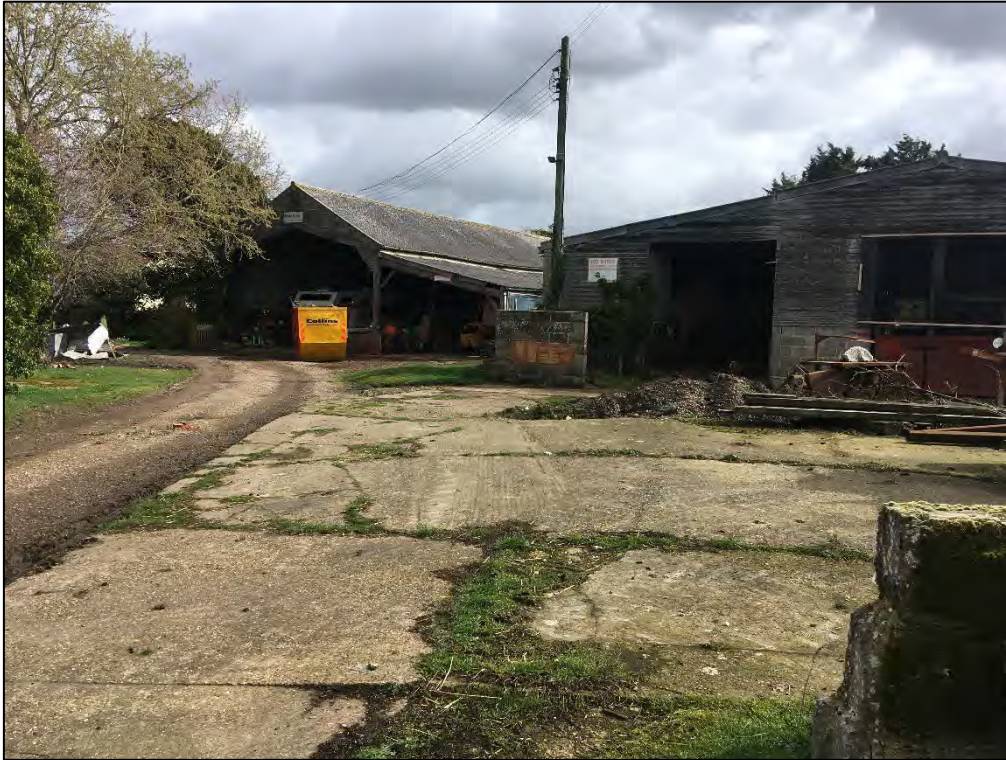
Photograph 33: Farm buildings to the south-east of the site.
