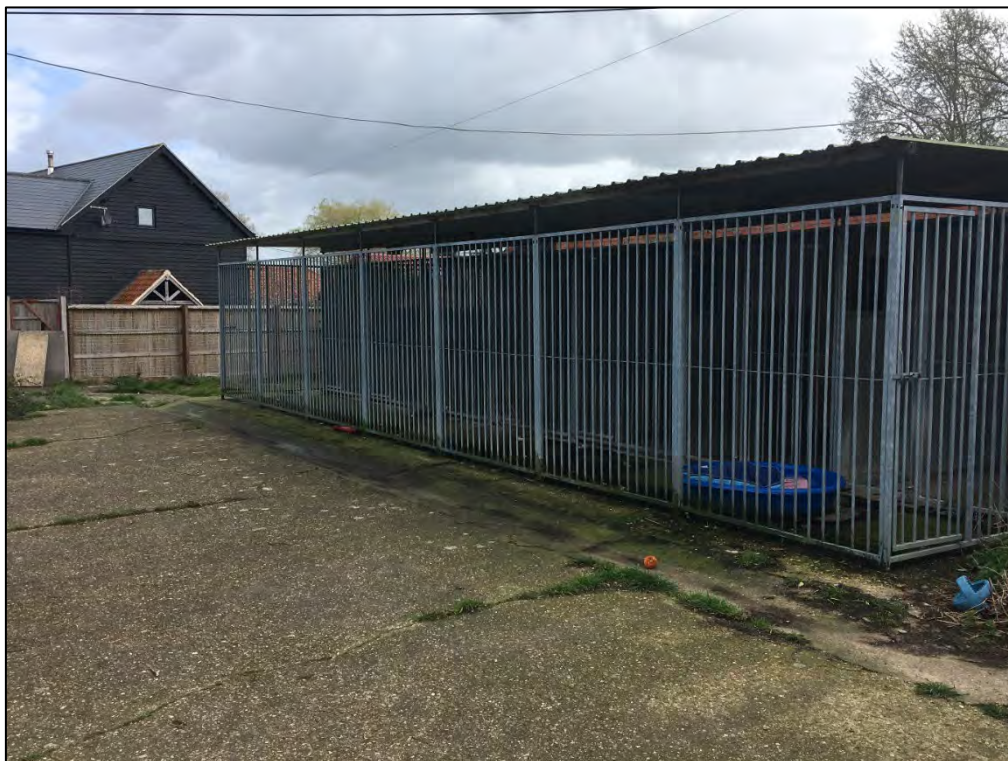
Photograph 10: Separate kennel building. (Building 3)
