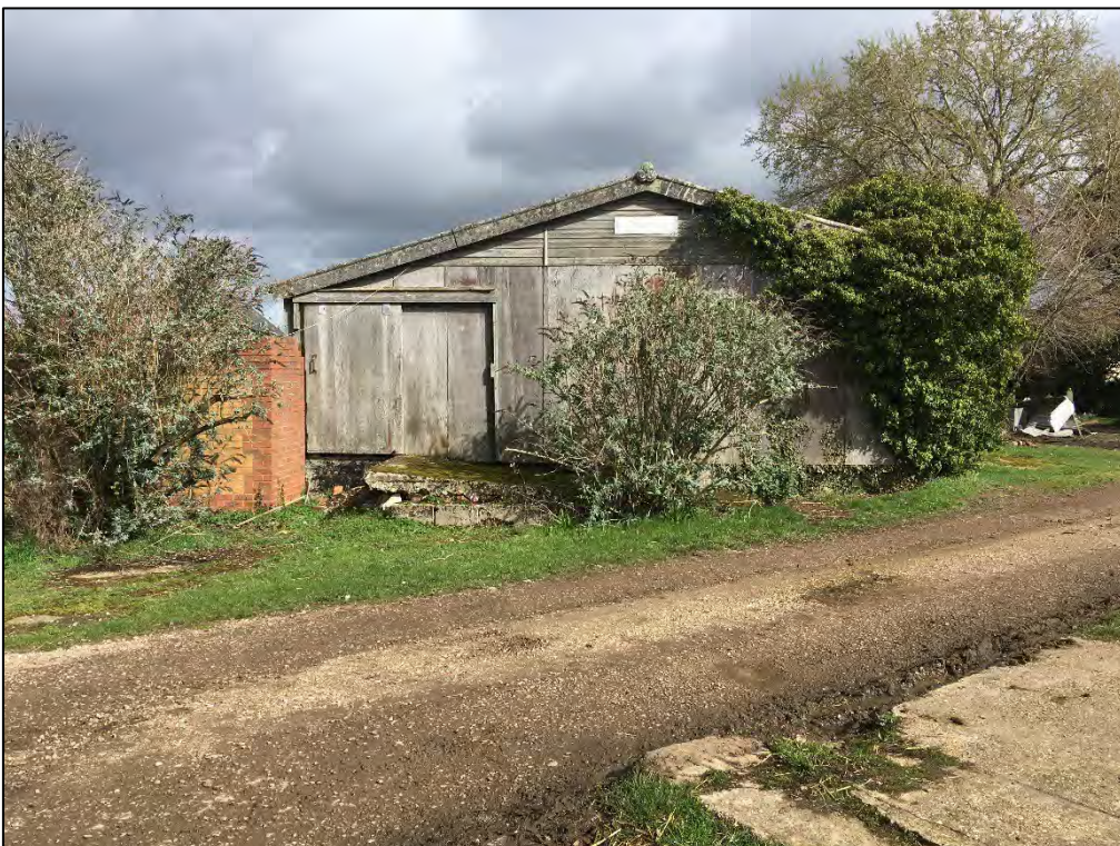
Photograph 4: The pig barn (Building 1).
