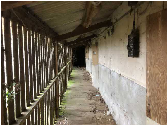
Interior of the former piggery.
