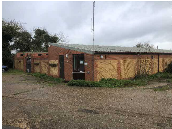
Exterior of the former boarding kennel buildings.
