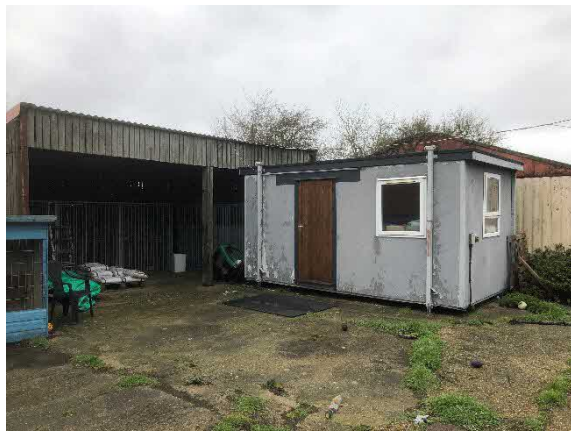
Storage buildings in the corner of the site.
