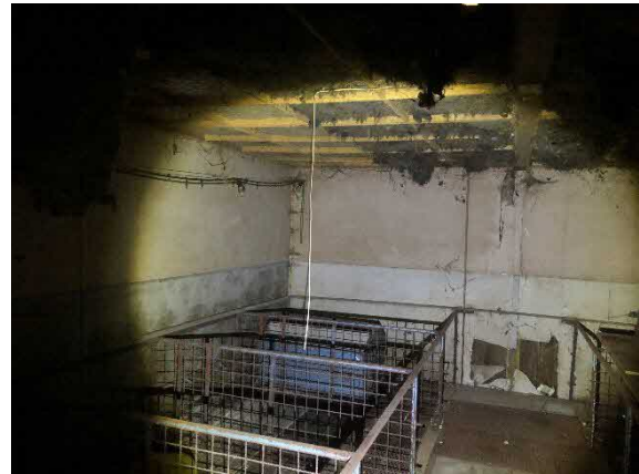
Interior of the former piggery.
