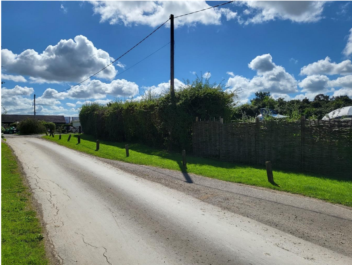
Existing Access Road to site – towards site turning, on right
