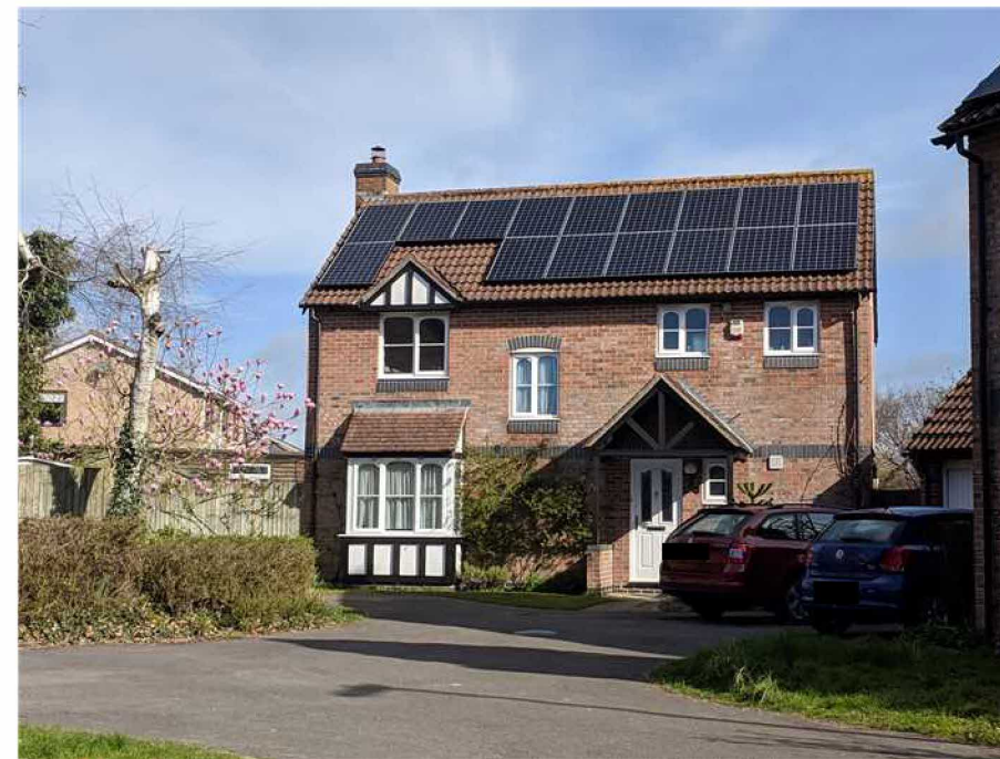
K2 tile mounting example installation
