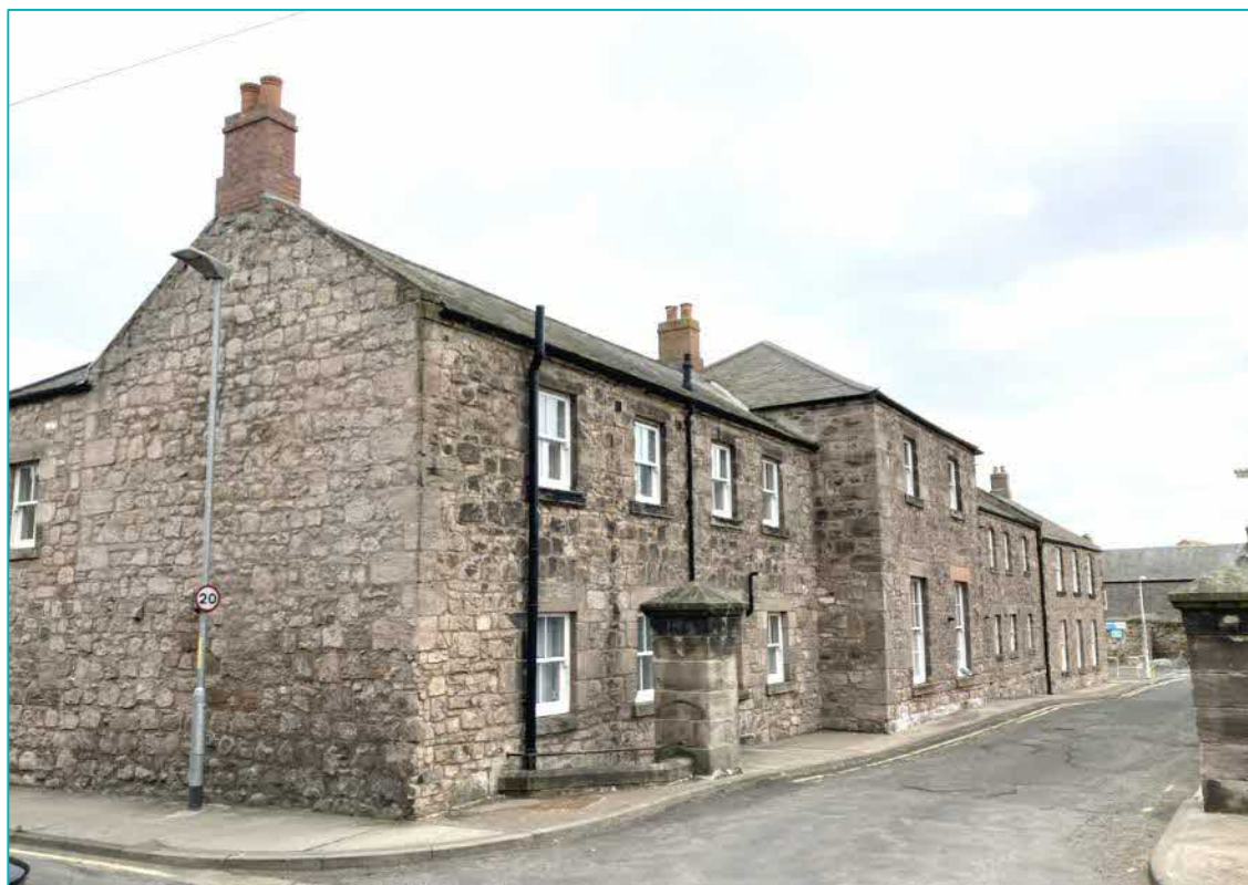
Figure 5.3 Former Berwick Union Workhouse (Non-Designated)
