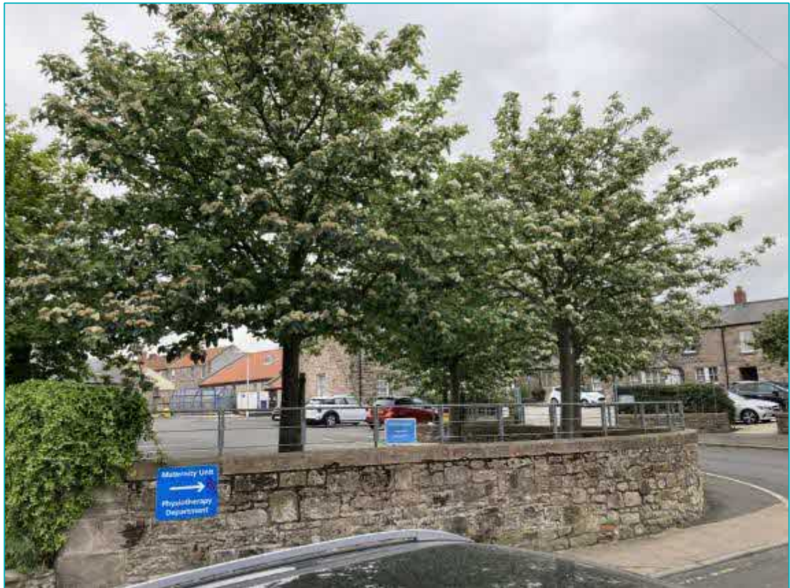
Figure 3.1 View of the site from Brucegate
