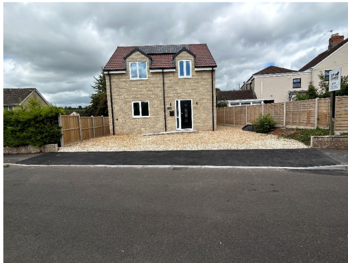
PHOTO 1 PROPERTY AND DRIVEWAY
