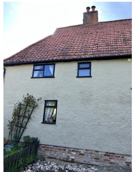
South east (rear) corner elevation
