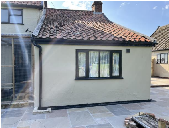
North east (rear) corner elevation
