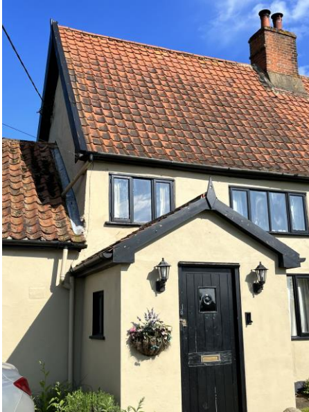
North west (front) corner elevation
